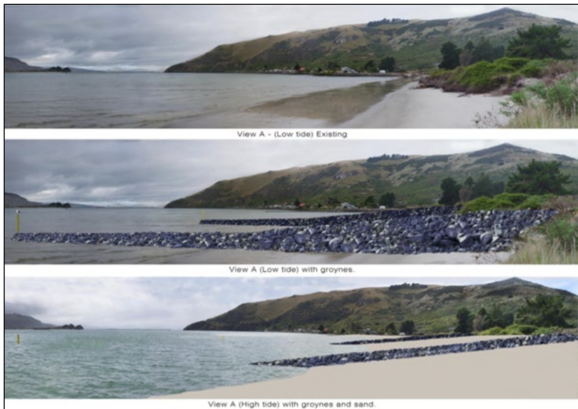
Figure 5: Visual representation of what the groynes will look like from the beach
