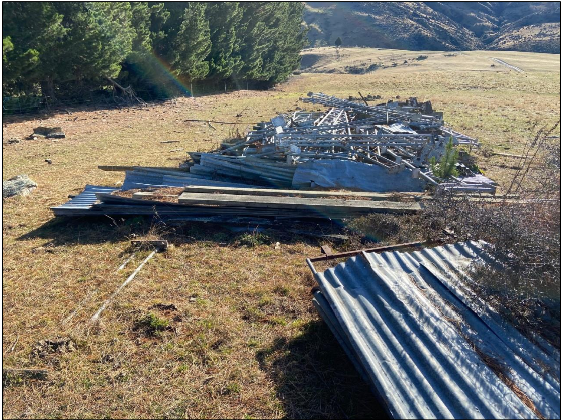
Figure 28: Habitat 12, buildings/farm litter in the north-eastern area of the PIA near existing woolshed.
