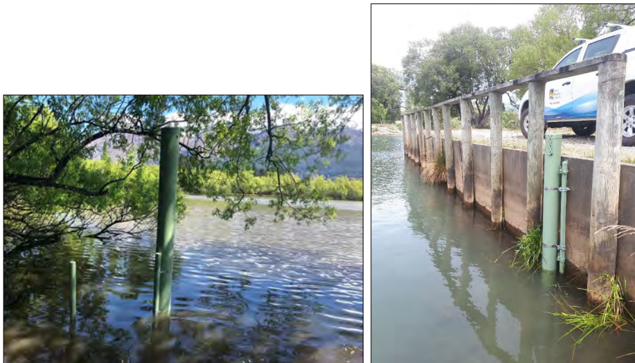
Figure 6: The recently installed water level monitors installed at the Glenorchy lagoon (6a, left) and the Glenorchy marina (6b, right). Data for both of these monitoring stations is available in near real-time on ORC's WaterInfo web page.
