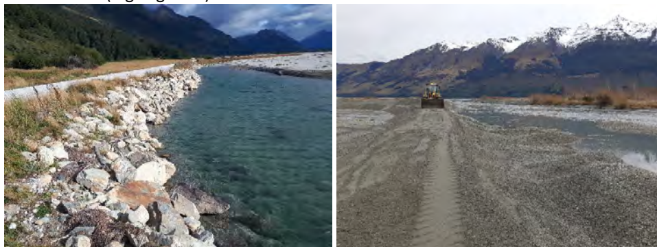
Figure 2: Examples of erosion protection and river management works. At left, rock armouring of a section of the Dart river banks at Kinloch Road (completed by QLDC). Right-hand image shows work undertaken by ORC at the Rees Delta to realign the main Rees River channel.
