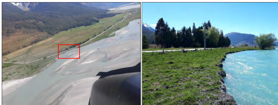
Figure 23: Aerial view (October 2020) of the Dart floodplain between the Dart Delta and Glacier Burn (left). The QLDC installed a section of rock armouring in this location in late 2020, with a financial contribution from ORC. The red outline indicates the location of the right-hand photograph, taken November 2020, and showing an area of active erosion which was rapidly progressing towards Kinloch Road.
