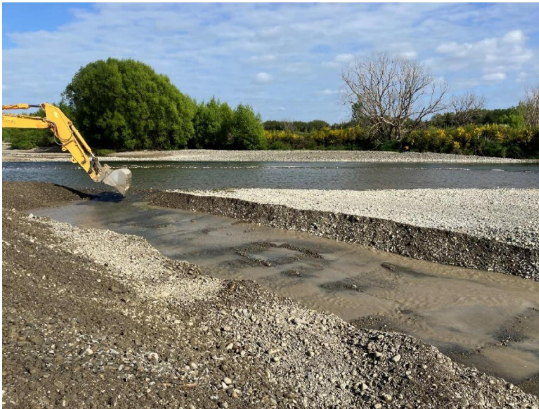
Figure 5: Example of works to create a diversion channel in Ashley River showing digger making final connection for a channel excavated in the dry riverbed (Source: Application CRC241485)
