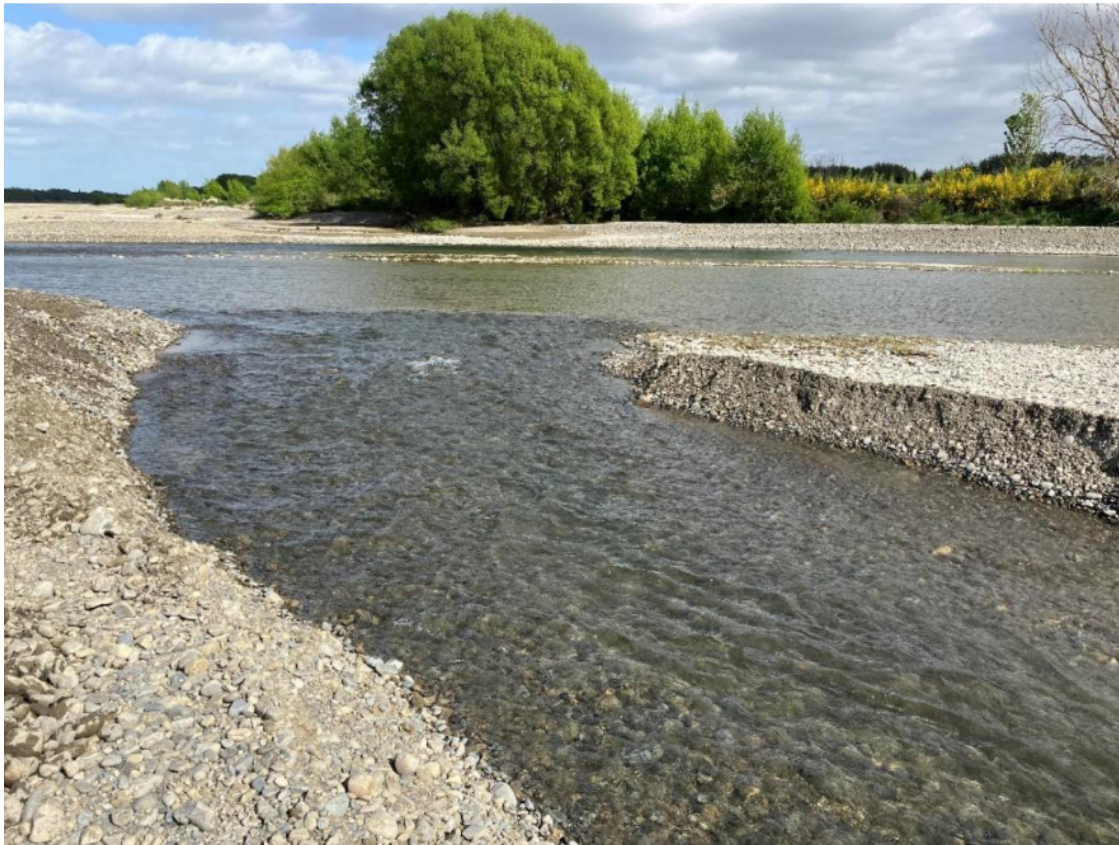
Figure 6: Example of works to create a diversion channel in Ashley River showing 10 minutes after the final cut was made (Source: Application CRC241485)
