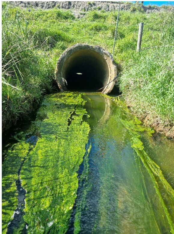
Figure 3: Culvert in between Christies Creek SW2b and Coal Creek SW3b.
