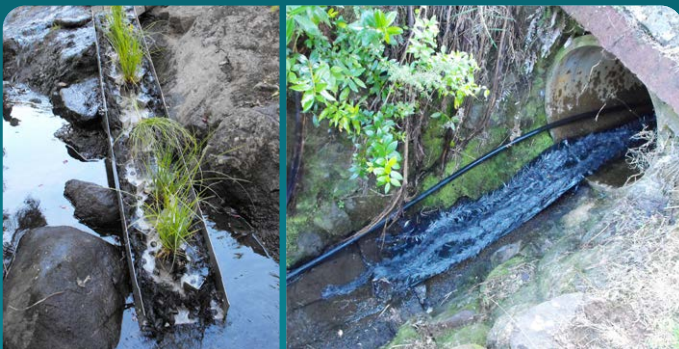
Figure 2. Fish passage enhancement including a ramp and spoiler baffles (left) and mussel spat ropes (right). Photo credit: Fish Ladder Solutions.
