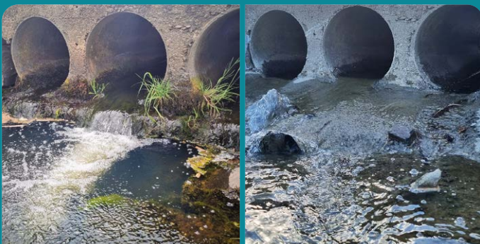
Figure 3. Before (left) and after (right) installation of a rock ramp to improve fish passage at the Patterson's Road ford. Photo credit: Matt Dale, Waterscape Connections.
