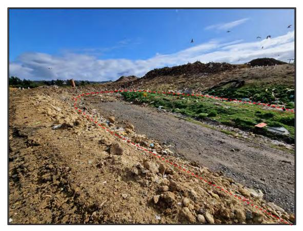
Photograph 14: Area prepared to receive asbestos materials to the west of the current tip face.
