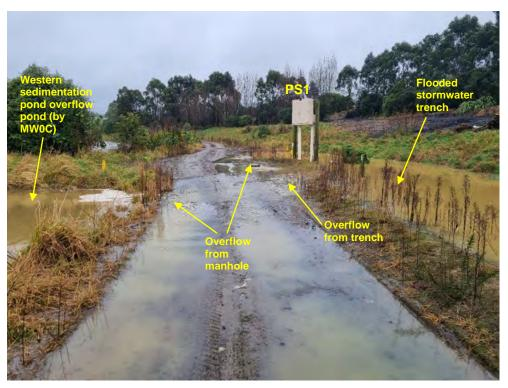
Photograph 6: Flooding of the leachate channel and overflow from PS1 into the W pond (by MW0C), looking north.
