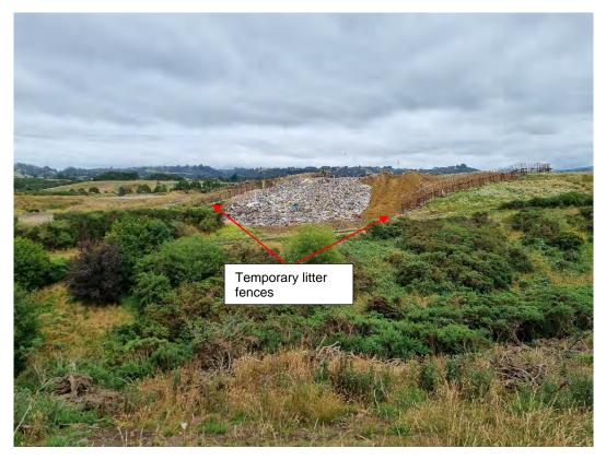
Photograph 5: View of the current tip face, indicating the location of the temporary litter fences looking north.
