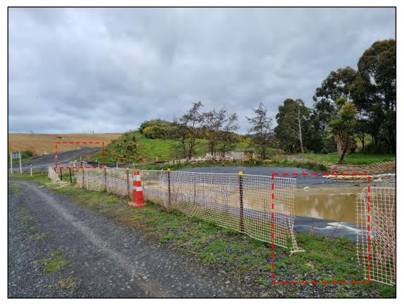
Photograph 3: Orange netting which requires replacement around the northern stormwater detention / sedimentation pond.
