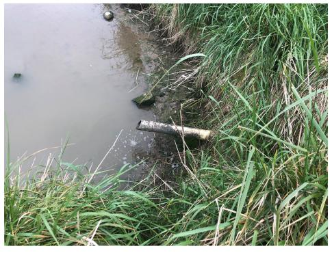
Photograph 2: 80mm PVC pipe outlet into the South Western Pond.
