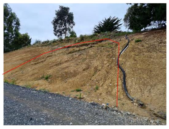
Photograph 7: Area of minor slump / erosion on the constructed road to the borrow pit.
