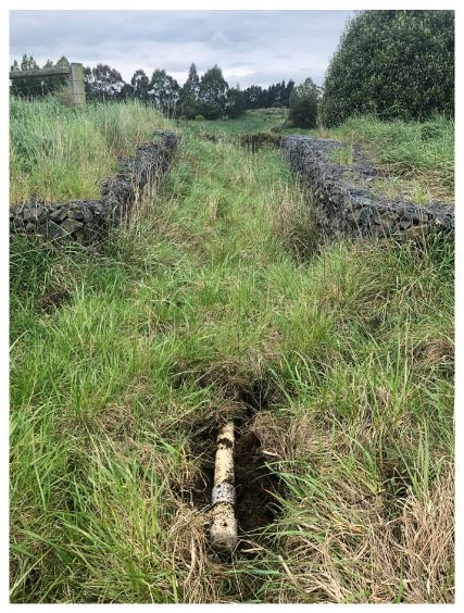
Photograph x: Capped Low level outlet under Western Sedimentation Pond weir
