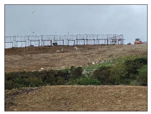
Photograph 4: Temporary fences have been moved but wind-blown waste has migrated beyond the fence boundaries.
