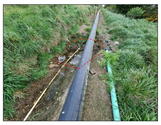
Photograph 1: A slight hole is present in the ground surface beneath the gas line to the east of line MWO.
