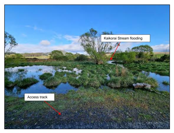
Photograph 15: Flooding associated with the Kaikorai Stream / Estuary mouth being blocked.
