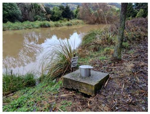
Photograph 20: Well MW7D's concrete base has been undercut and is unstable.
