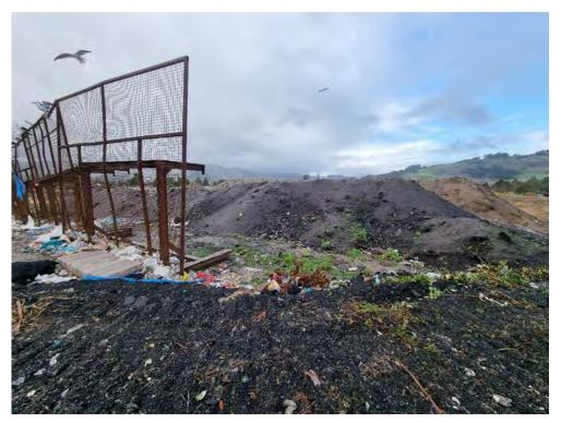
Photograph 16:The litter fence and stockpiled material within the vicinity of the tip face which will be utilised as final capping material.
