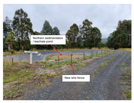
Photograph 1: A new barrier has been constructed around the northern sedimentation / leachate pond.
