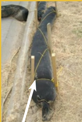
Tie and peg down to secure
