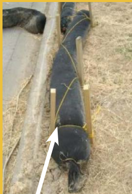
Tie and peg down to secure
