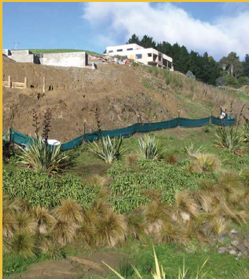
Silt fence and vegetation buffer
