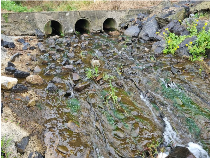
Figure 36. The established rock ramp at Brooklands Road ford.
