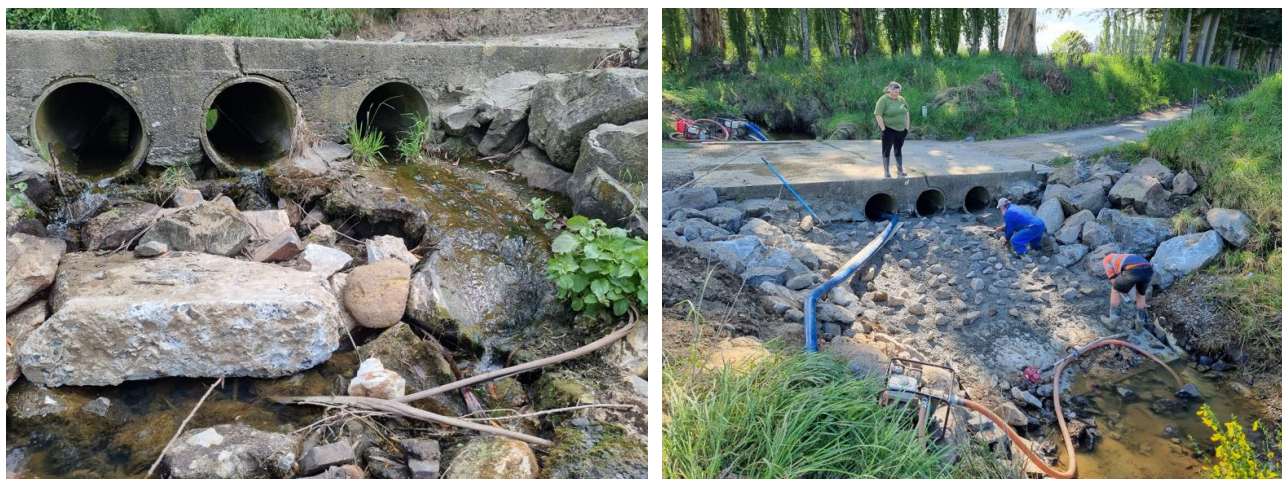
Figure 35. The Brooklands Road ford before (left image) and during (right image) construction of a rock ramp to improve fish passage.
