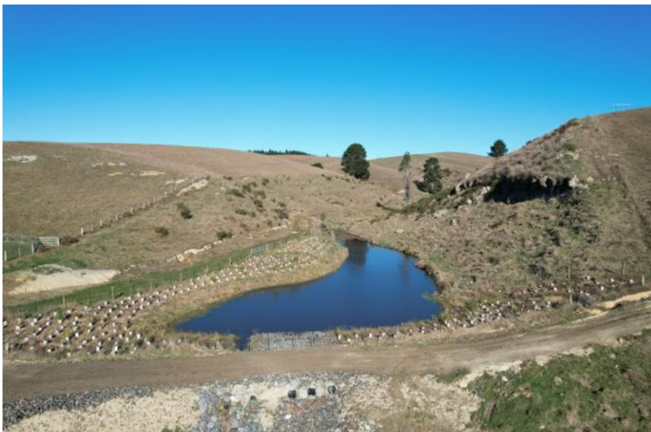
Figure 32. One of the series of sediment traps (shown by the blue ovals in Figure 31) established in June 2024, part way through the monitoring period, in the watercourse within an erosion prone gully on farmland discharging into Te Hikapupu/Pleasant River.
