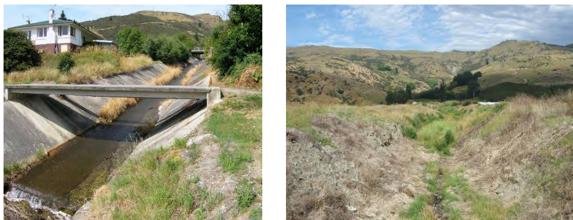
Figure 9: Different types of artificial channel at Roxburgh. LEFT: A steep concrete-lined channel conveys Reservoir Creek down its equilibrium to slightly terraced fan in the Roxburgh urban area (Opus photo, Jan 2009). RIGHT: Gravel embankments up to 4 m high constrain the course of Slaughterhouse Creek on the centre of its equilibrium to aggradational fan, north of Roxburgh. The gradient of its channel is much less than that of Reservoir Creek, and the Slaughterhouse Creek channel therefore has a correspondingly lesser ability to transport coarse sediment such as gravel or boulders (GNS Science photo, Jan 2009).
