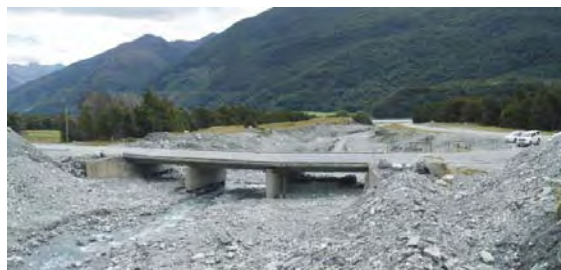
Pipson Creek fan at the highway bridge. Large gravel embankments, constructed from debris that has choked the channel, currently direct the active channel straight down the fan to the Makarora River ( GNS Science photo, Jan 2009 )
