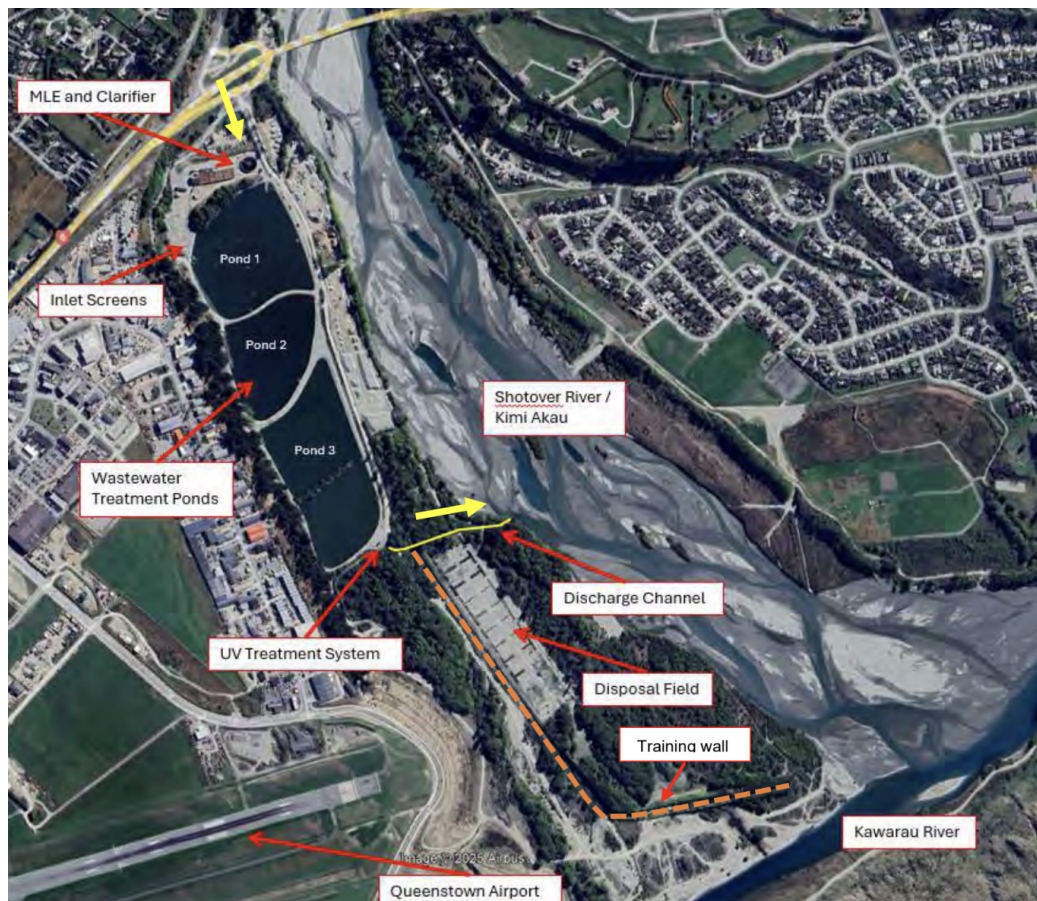
Figure 1. Map showing proximity of disposal field to the airport runway 2
