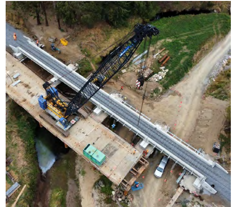
Bridge 194 Main South Line across Pleasant River at Goodwood
