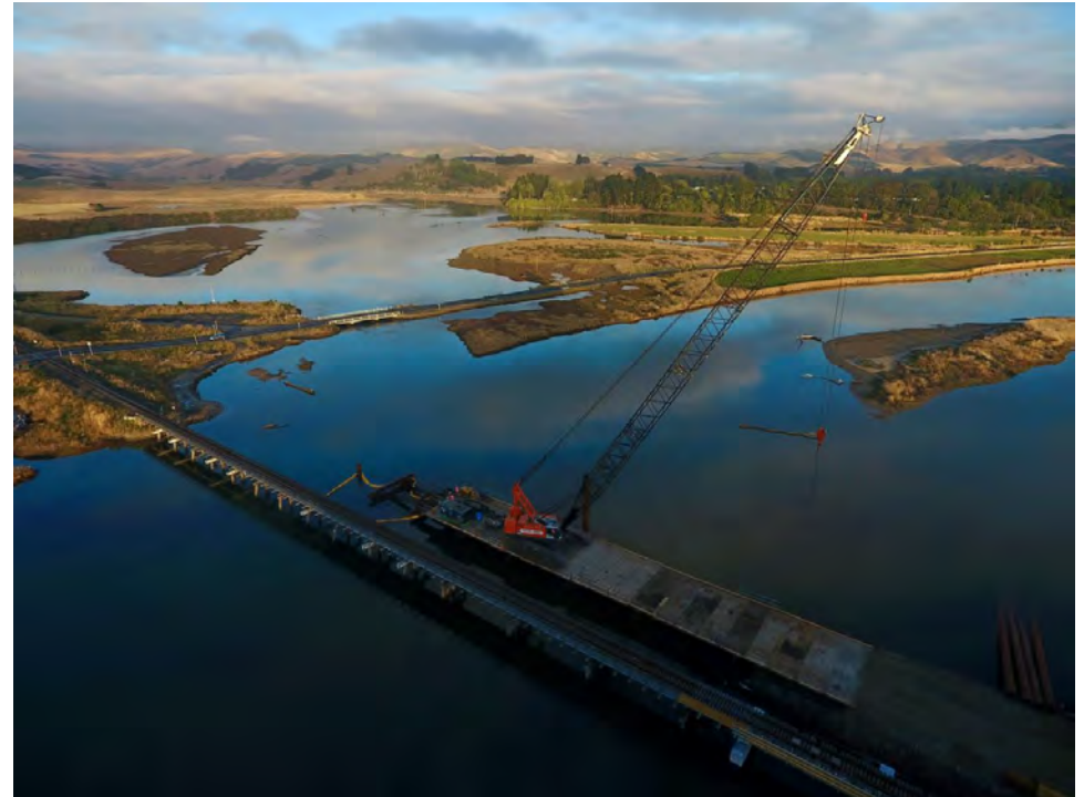
Bridge 202 on MSL at Waikouaiti during RNIP 1 works in 2022
