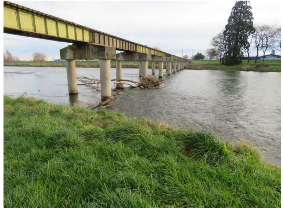
Bridge 348 on MSL at Gore
