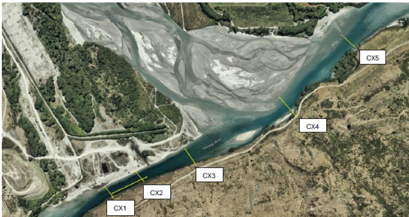
Figure 3.14 Kawarau River surveyed transect locations, as indicated by yellow lines with cross-sections numbered. Longitudinal profile indicated between cross-sections CX1 and CX2 (ESNZ, 2026)
