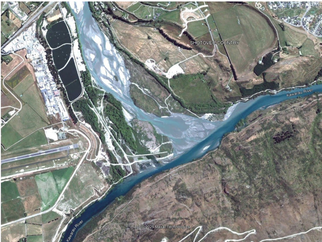
Figure 3.5 Aerial image taken 21 January 2013, shortly after flood training wall construction
