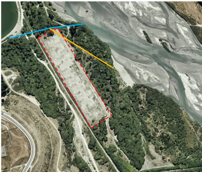
Figure 2.1 Approximate location of first drain (orange) and second drain (blue) where treated wastewater was discharge to the Kimiākau/Shotover River. Approximate location of the DaD field is shown by dashed red line.
