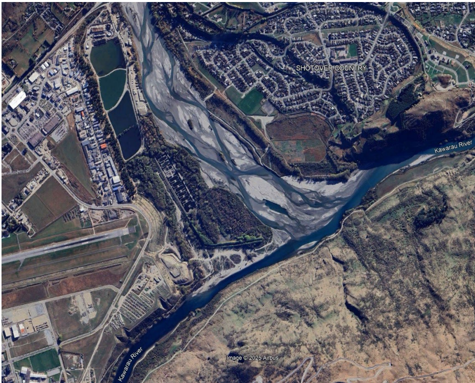
Figure 3.6 Aerial image taken 11 May 2024, post flood training wall construction
