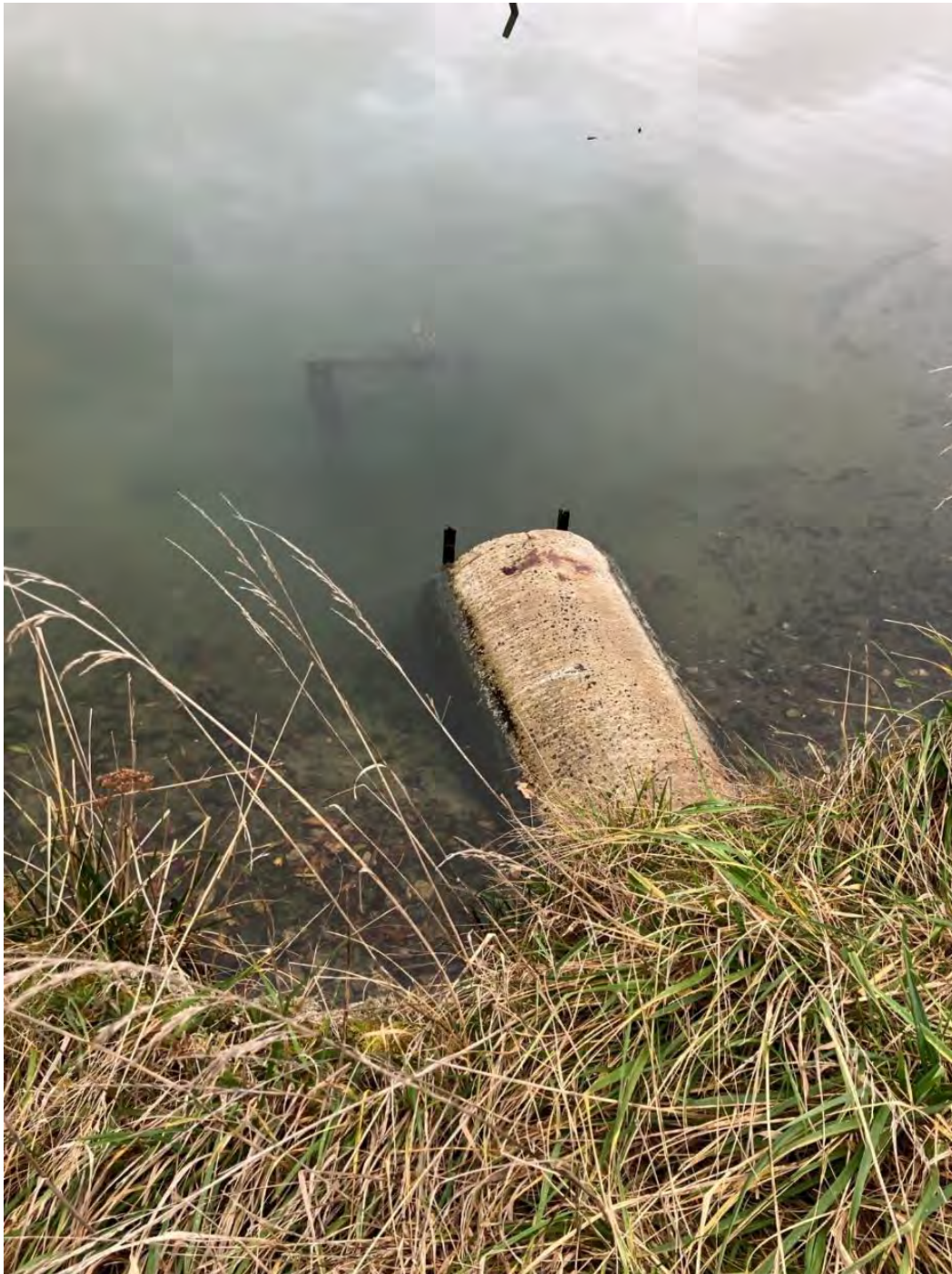
Figure 5: View of existing culvert through causeway into southern lagoon
