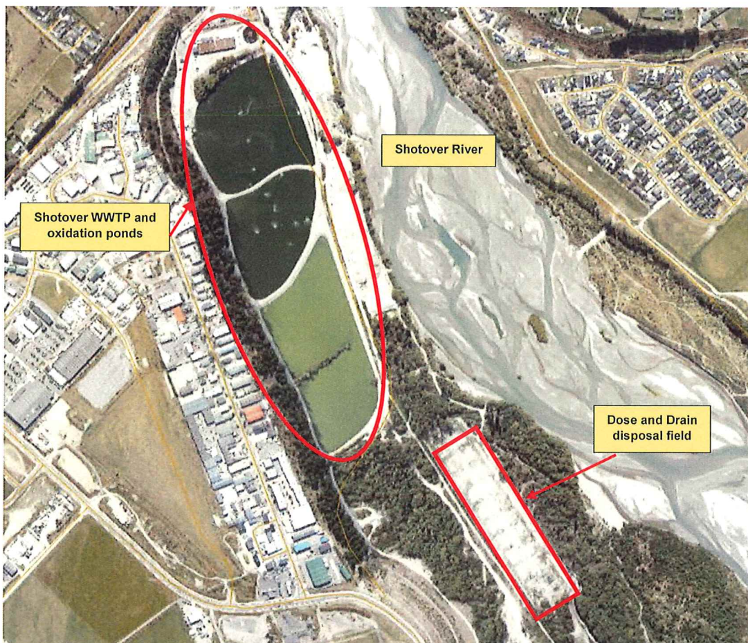
Figure 2-1: Aerial overview of the Shotover WWTP.
