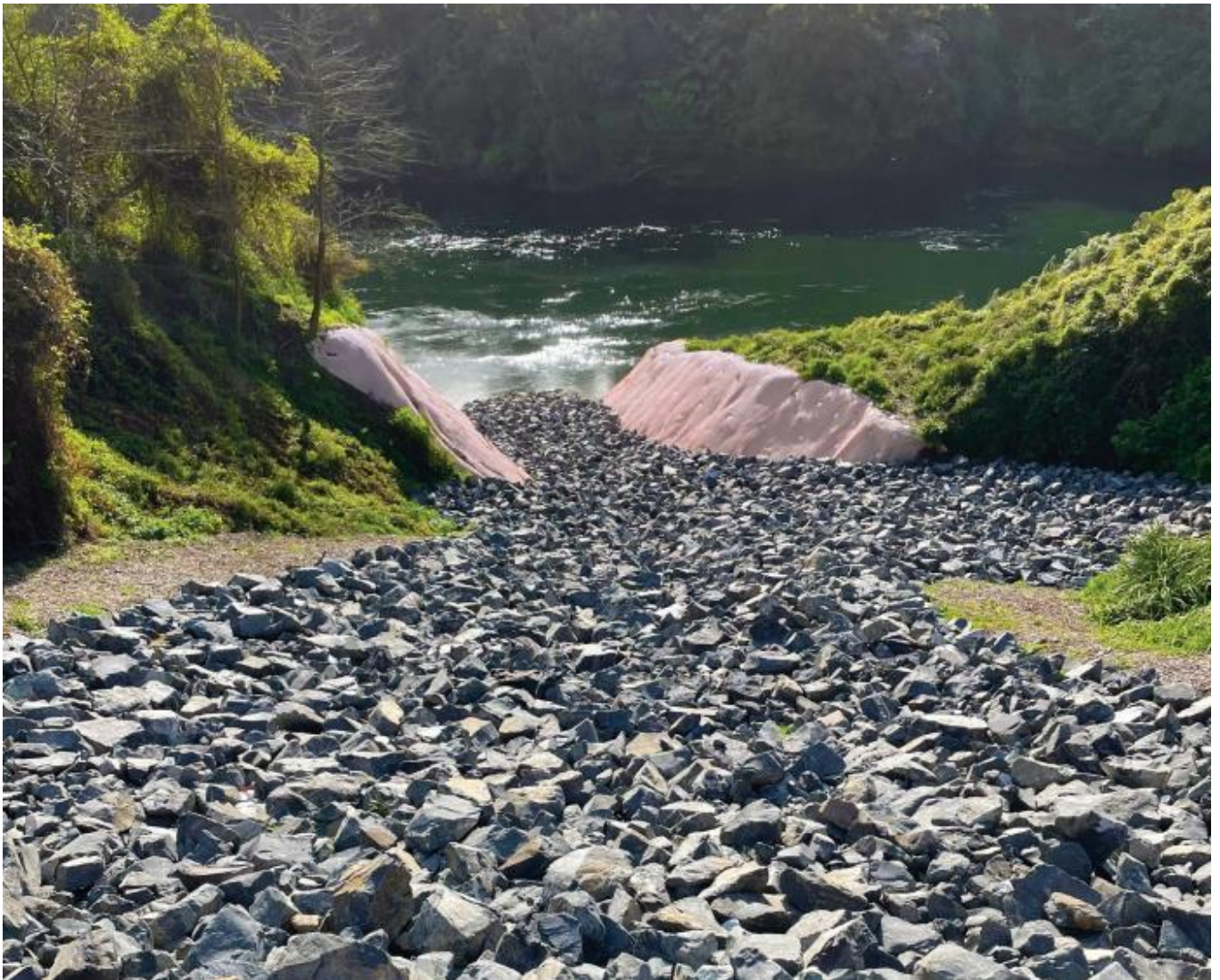
Figure 9 Example land flow path to river at Cambridge WWTP to Waikato River
