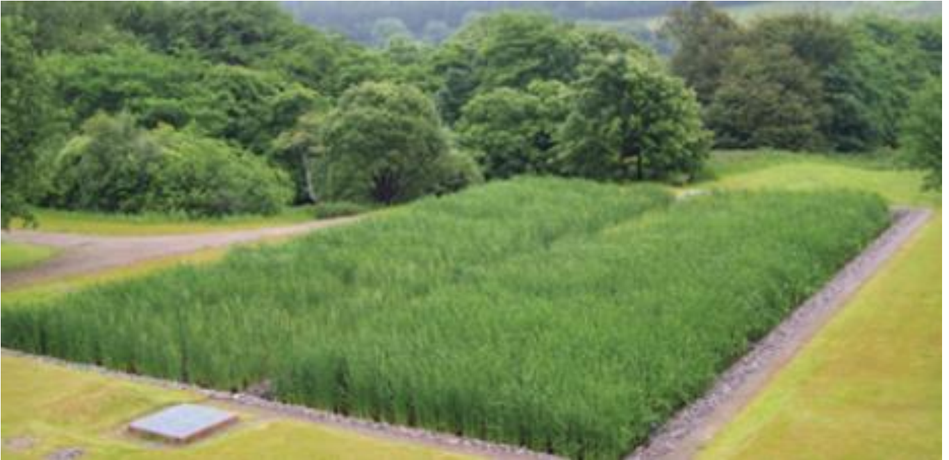
Figure 15 Example subsurface wetlands for WWTP tertiary treatment overseas.
