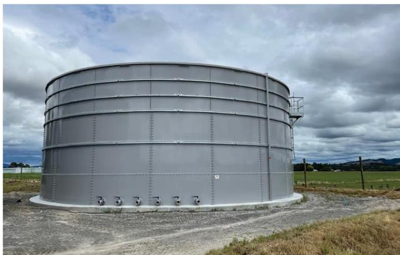
Figure 19 Example of bolted steel storage tank (Reliant Solutions)
