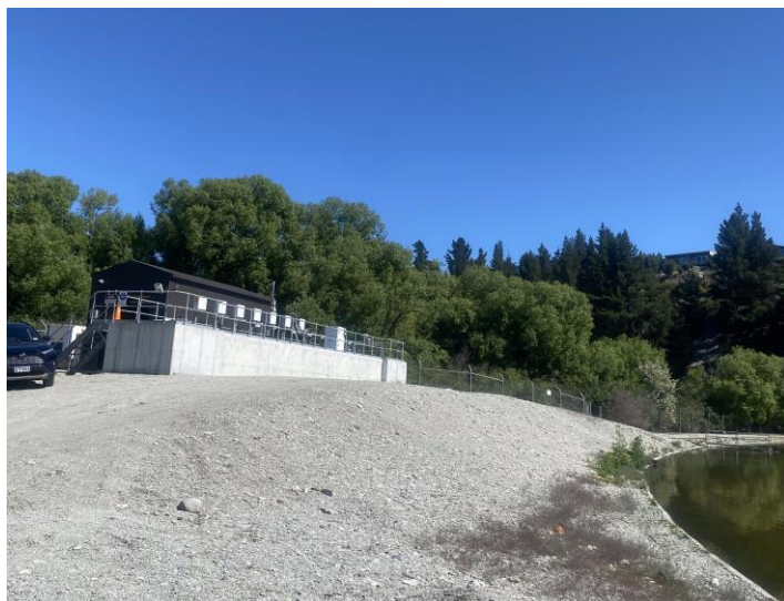
Figure 3 Current UV site at Shotover WWTP, photo taken 2024
