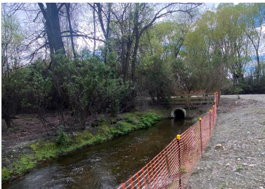
Figure 23 Discharge channel, October 2025, (prior to planned installation of permanent fencing).
