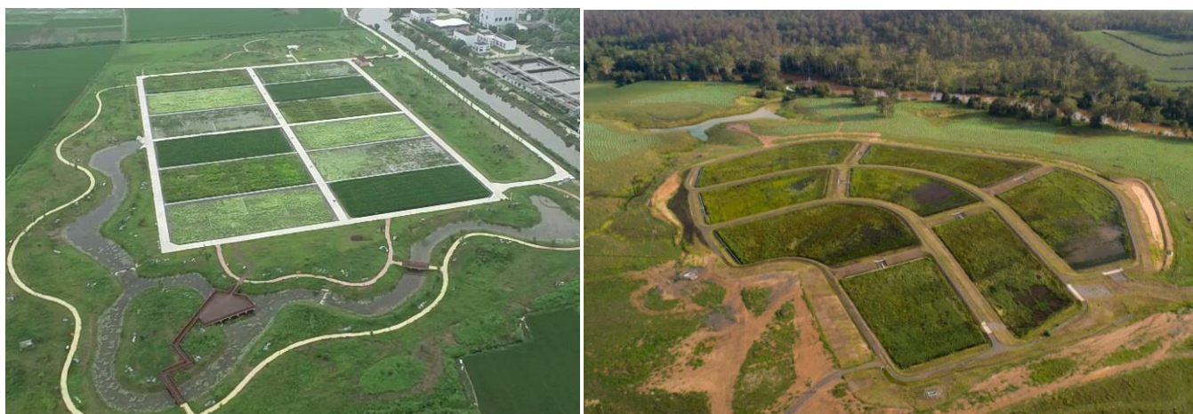
Figure 16 Two subsurface wetland examples - Jian Li City (2.4ha) in China and Cedar Grove WWTP (7.7ha) in Queensland
