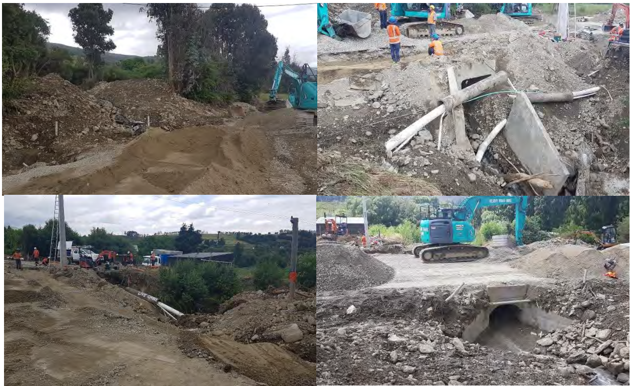
Figure 15: SH8 culvert damage at Pumpstation Creek as a result of the 2017 debris flood.
