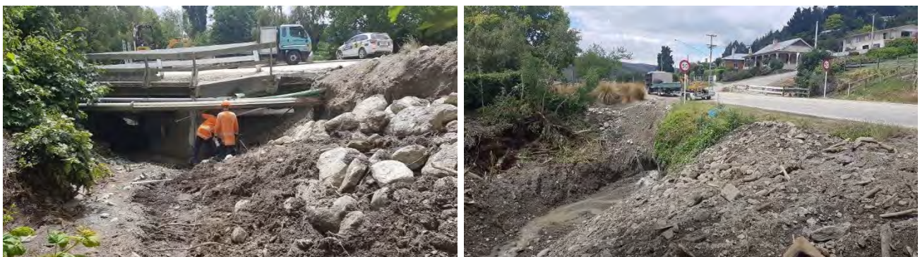
Figure 13: Photos of the Edinburgh Street culvert along SH8 following a debris flood.
