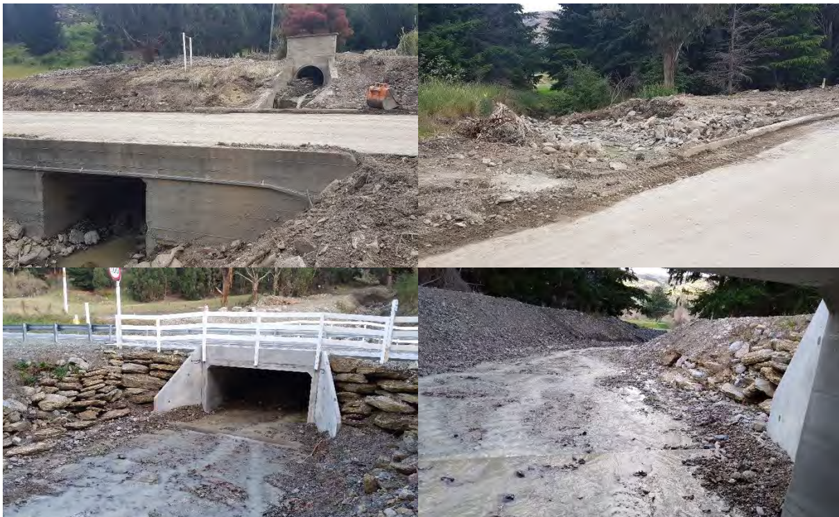
Figure 12: Top left and top right: The 2017 debris flood at SH8 crossing of Golf Course Creek. Bottom left and bottom right: The new culvert at Golf Course Creek pictured in 2023.
