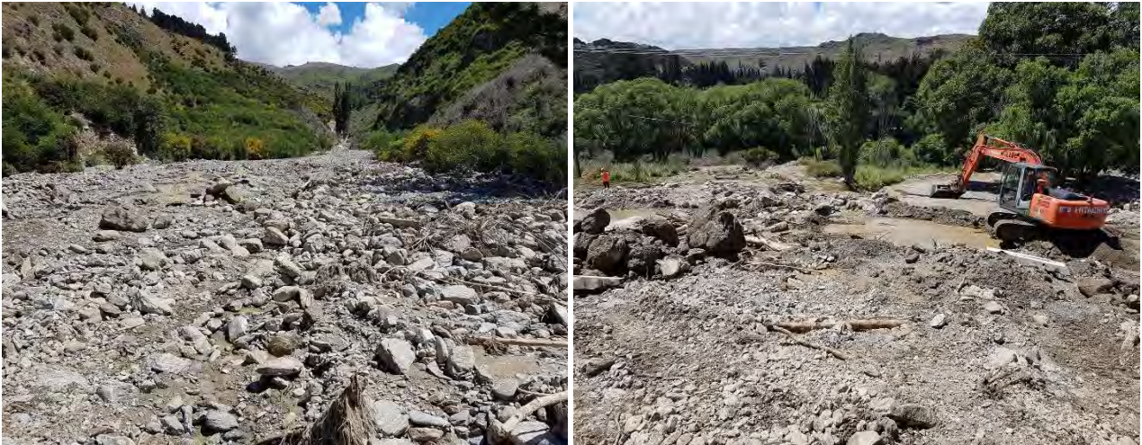
Figure 10: Left: Debris flood deposit in Black Jacks Creek upstream of SH8 November 2017. Right: Debris flood deposit on SH8 from Black Jacks catchment. The surface of the road has been exposed by the excavator.
