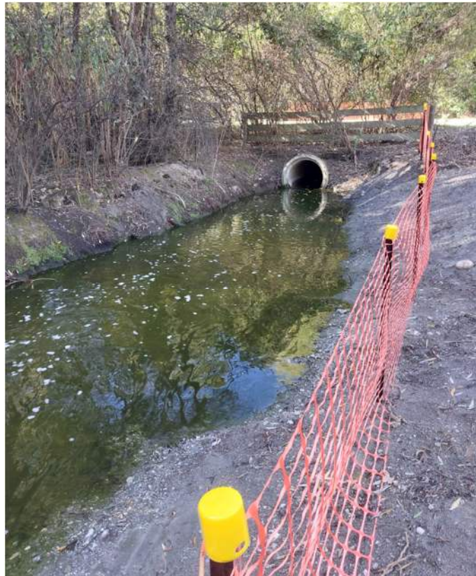
Figure 41: Example of temporary safety fencing around discharge channel, along with culvert and pre-existing fencing
