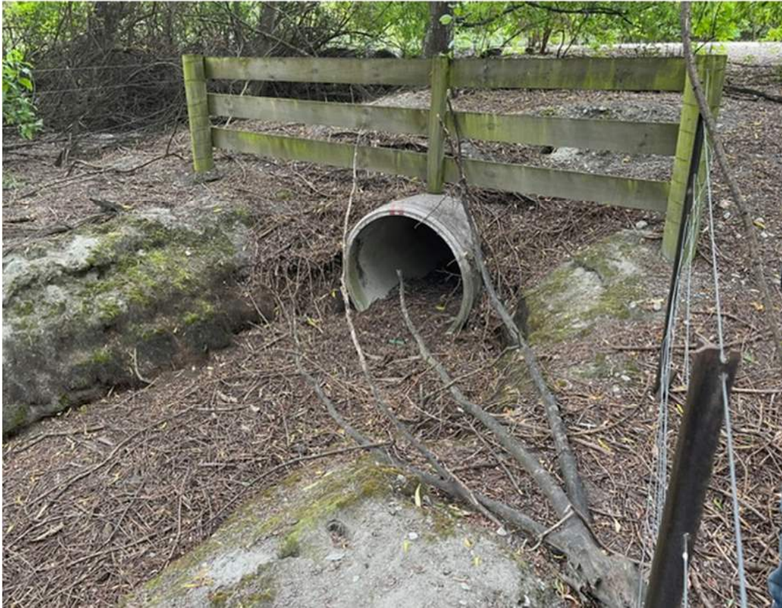
Figure 23 Existing culvert along previous channel
