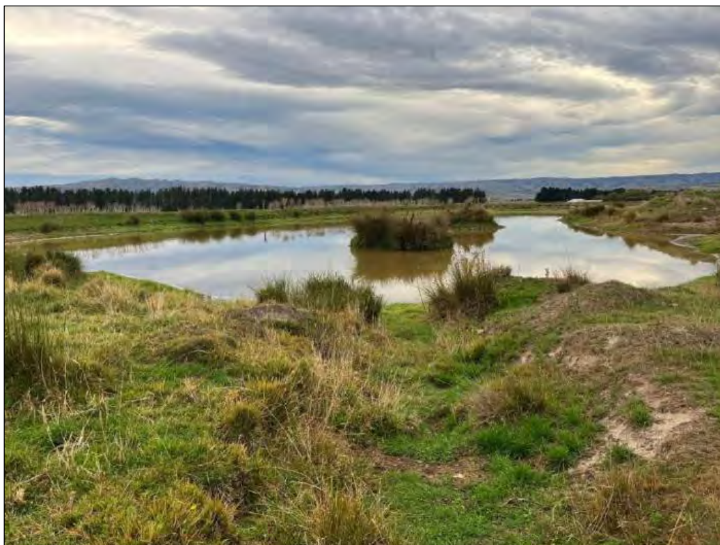
Figure 26: Smaller Storage Pond looking South
