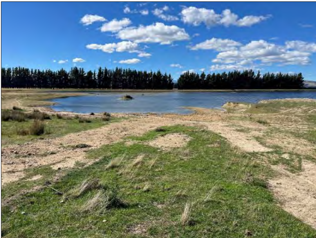
Figure 2.10: Main Storage Dam for Irrigation Looking East
