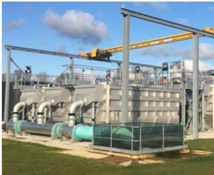
Figure 6: Example figure of tertiary filter installation (online photo, from WaterProject)
