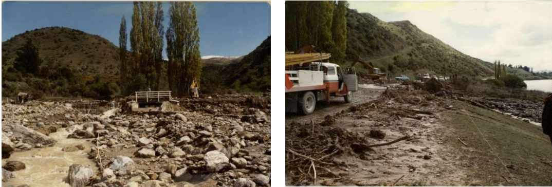
Figure 10. Sedimentation on the lower reach of Black Jacks Creek – 15 October 1978. Left photo is looking upstream to the culvert under SH8 and the right photo is looking along SH8 towards Roxburgh Township (OCB photos).
