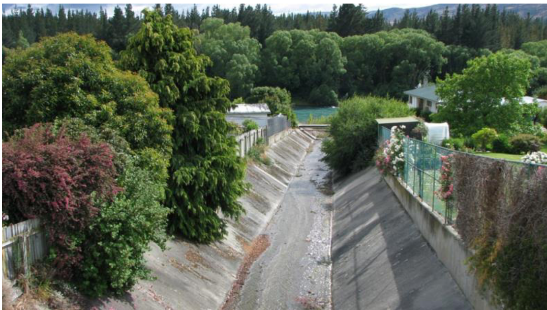
Figure 9. Concrete lined channel in the downstream section of Reservoir Creek (2009, ORC staff photo).
