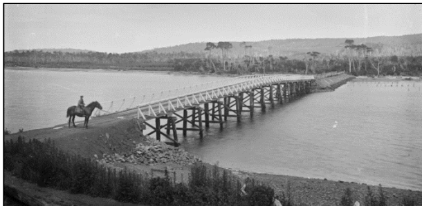
Hinahina Road bridge (1926) looking south, with native vegetation cover on the estuary margin (source: Alexander Turnbull Library, Wellington, New Zealand).
