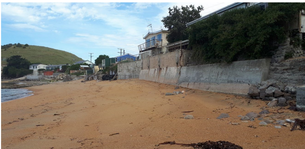
Figure 5: Privately constructed seawalls along Kaika Beach, north of Dunedin.
