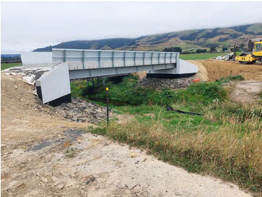
Figure 1. Completed Bridge 14 replacement.
