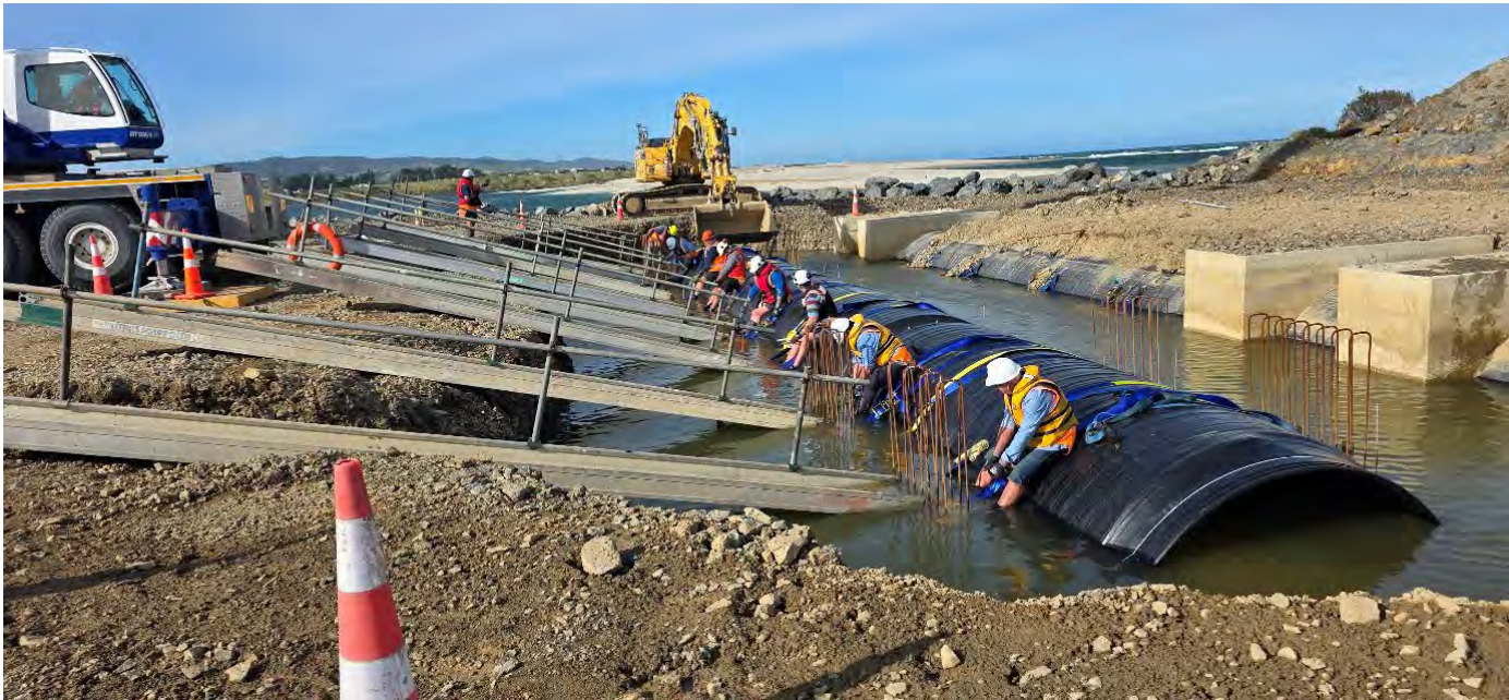
Figure 4. One of the 6 new culverts is ratcheted into place before the form work for the concrete anchor is formed and poured.
