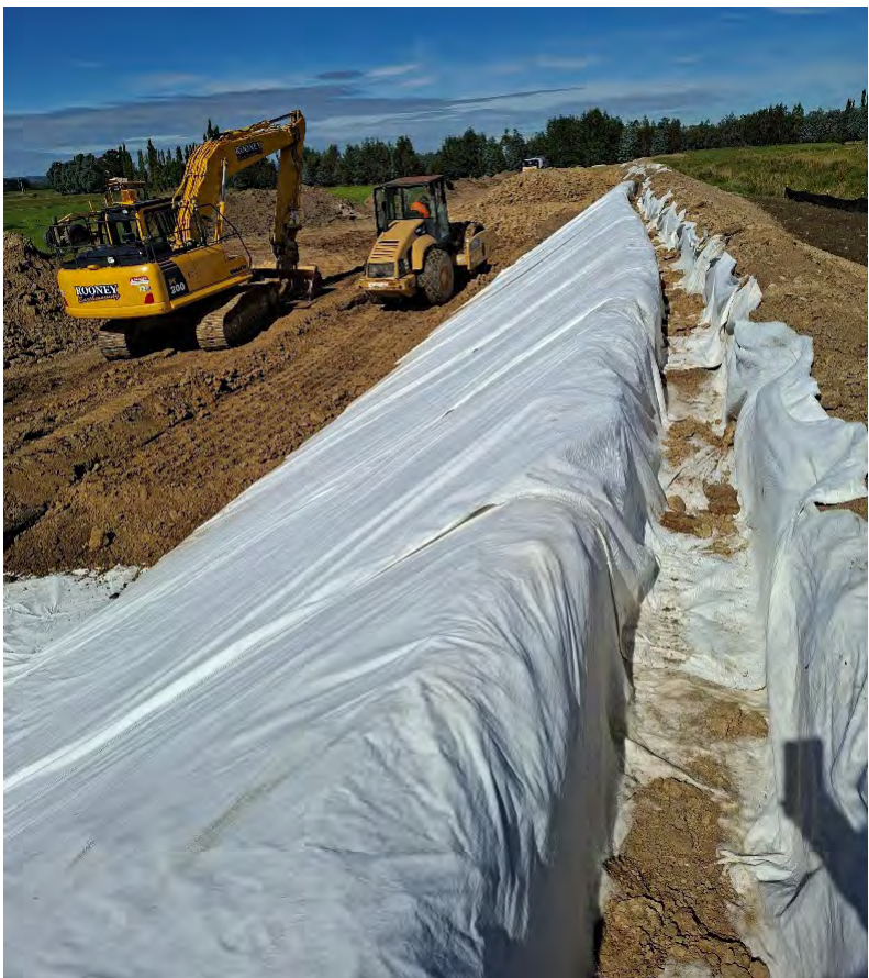
Figure 2. Contractor working on the new floodbank at the Woodside end of the Contour Channel.
