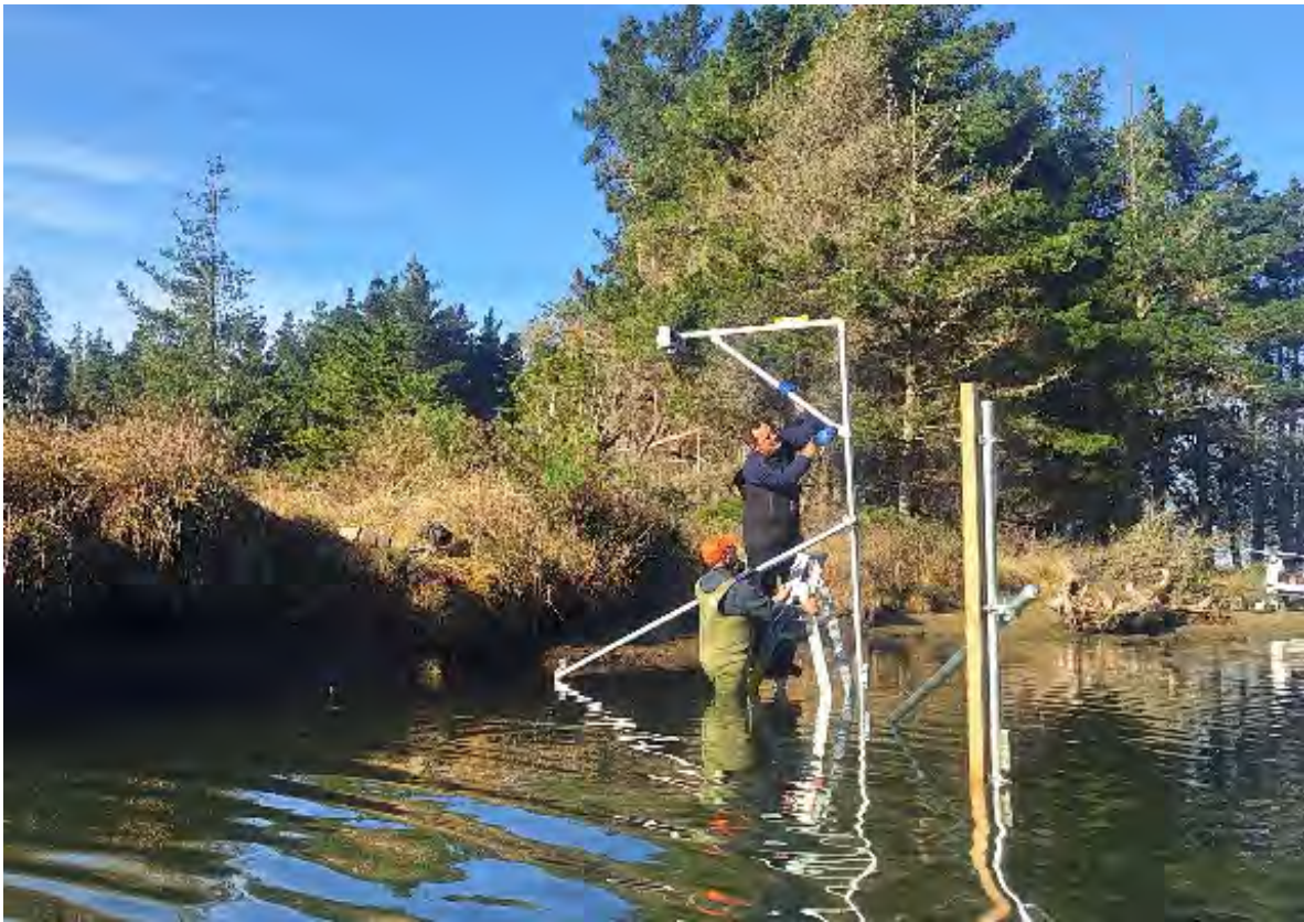
Figure 6. Environmental Monitoring staff installing one of the new level sensors.
