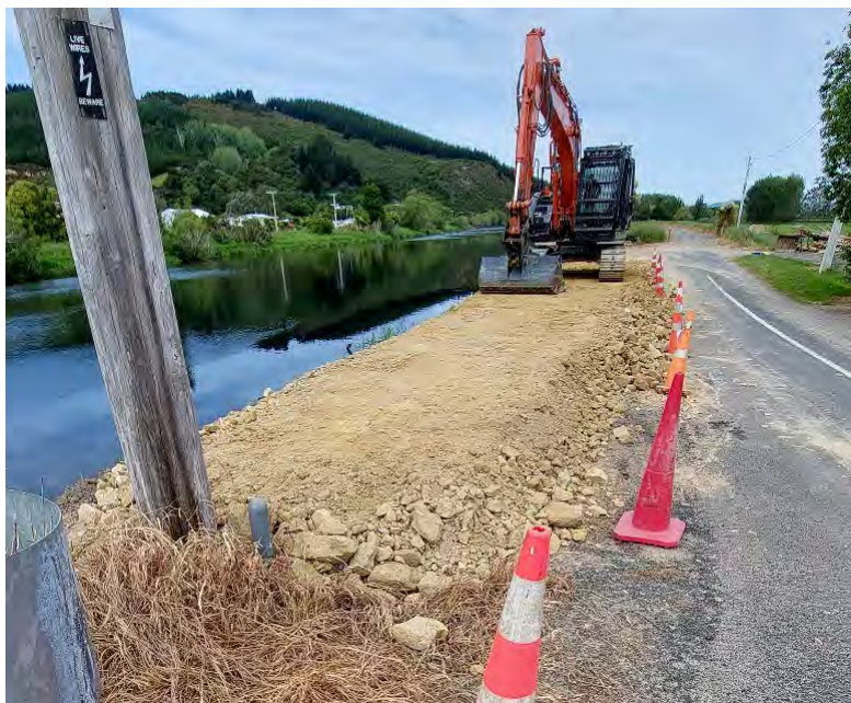
Figure 7. Floodbank being remade after the bites have been repaired.
