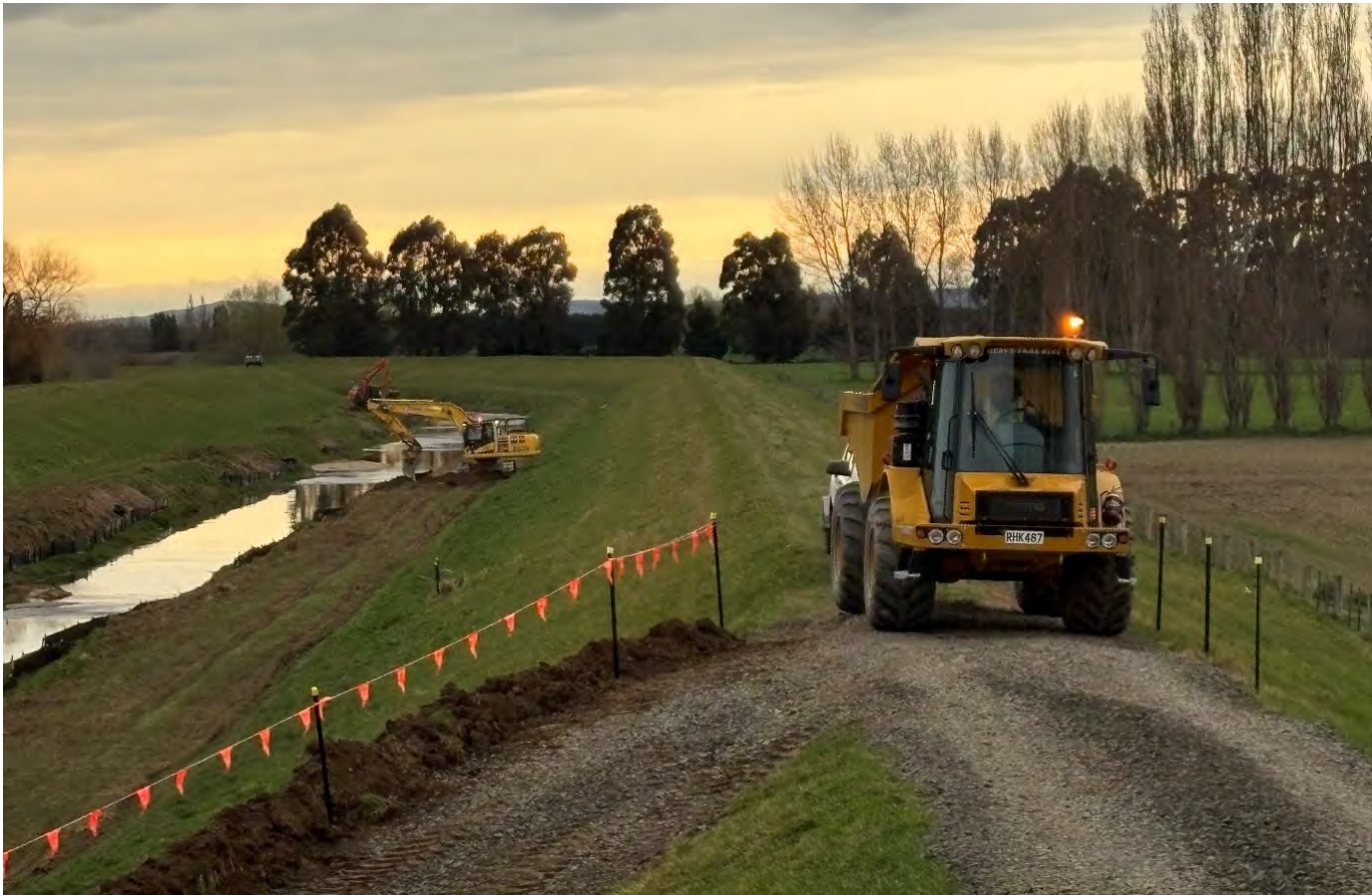
Figure 5. Contractor working on the berm at the Confluence end of the Silver Stream.
