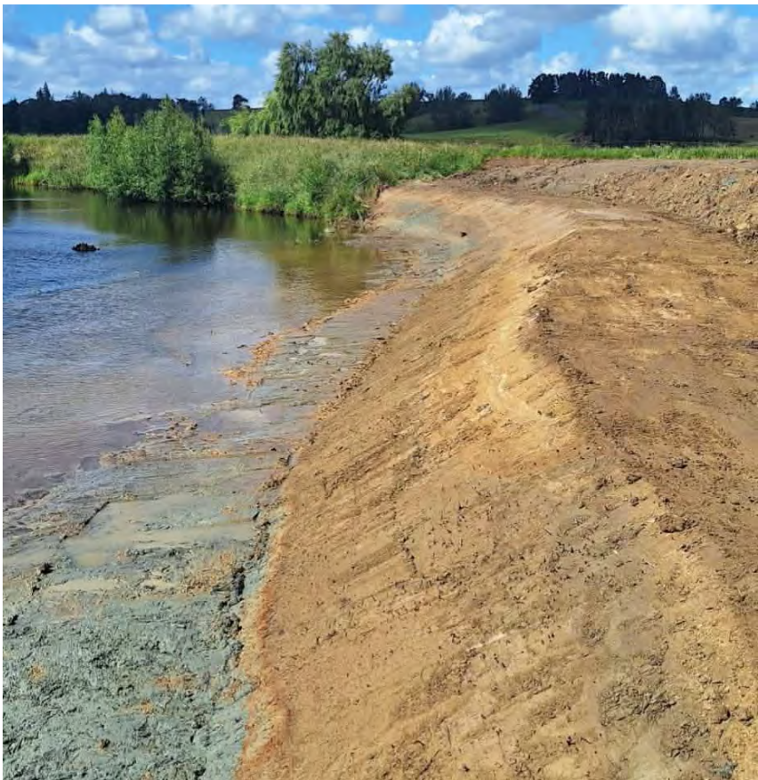
Figure 2. Bites removed and the berm battered back to design level.
