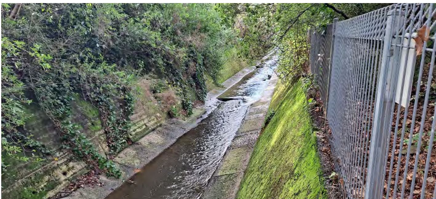
Figure 1. Typical sections of the Lindsay Creek channel in North East Valley (all looking upstream). Note the narrowness of the channel, the steepness of the right bank and the proximity of the houses and residential activities at many locations along the stream channel. The concrete channel lining and floodwall are ORC assets, some infrastructure is also owned, controlled and maintained by Dunedin City Council and adjacent private landowners.
