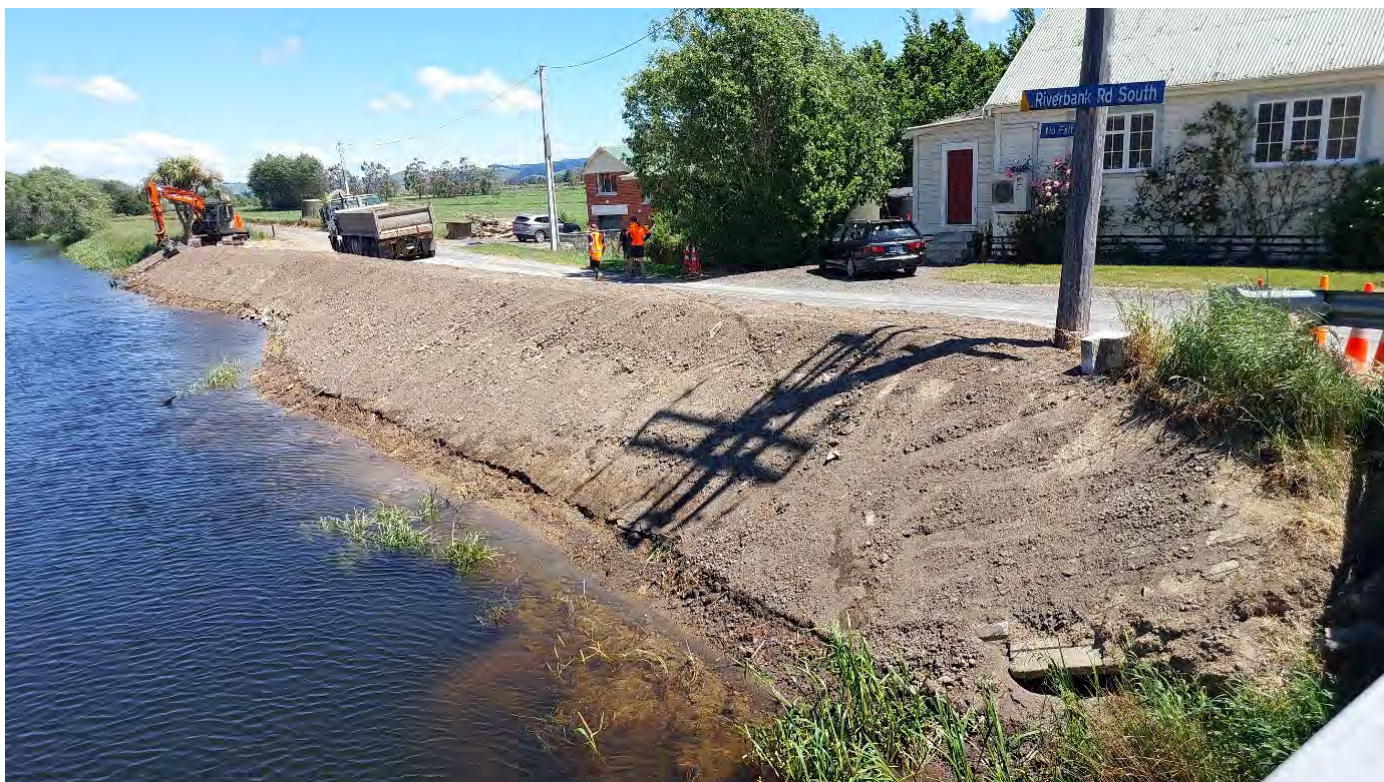
Figure 8. Contractor adding the final layer of dressing before seeding.
