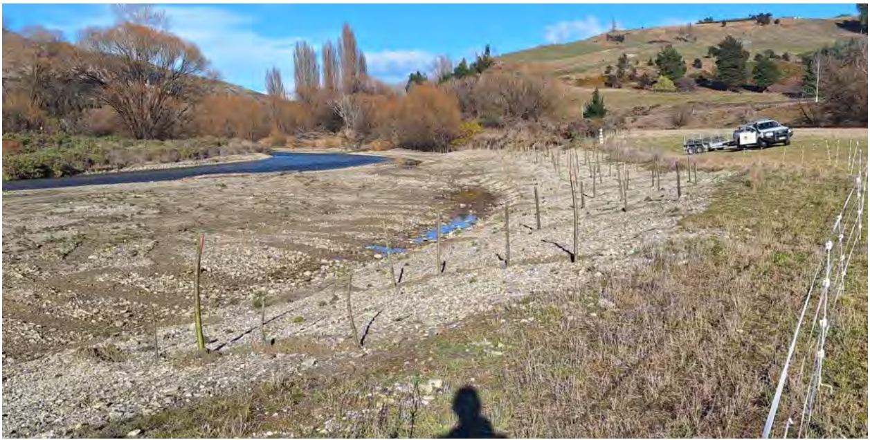
Figure 5. Bite repairs are complete and new trees planted to protect the road.
