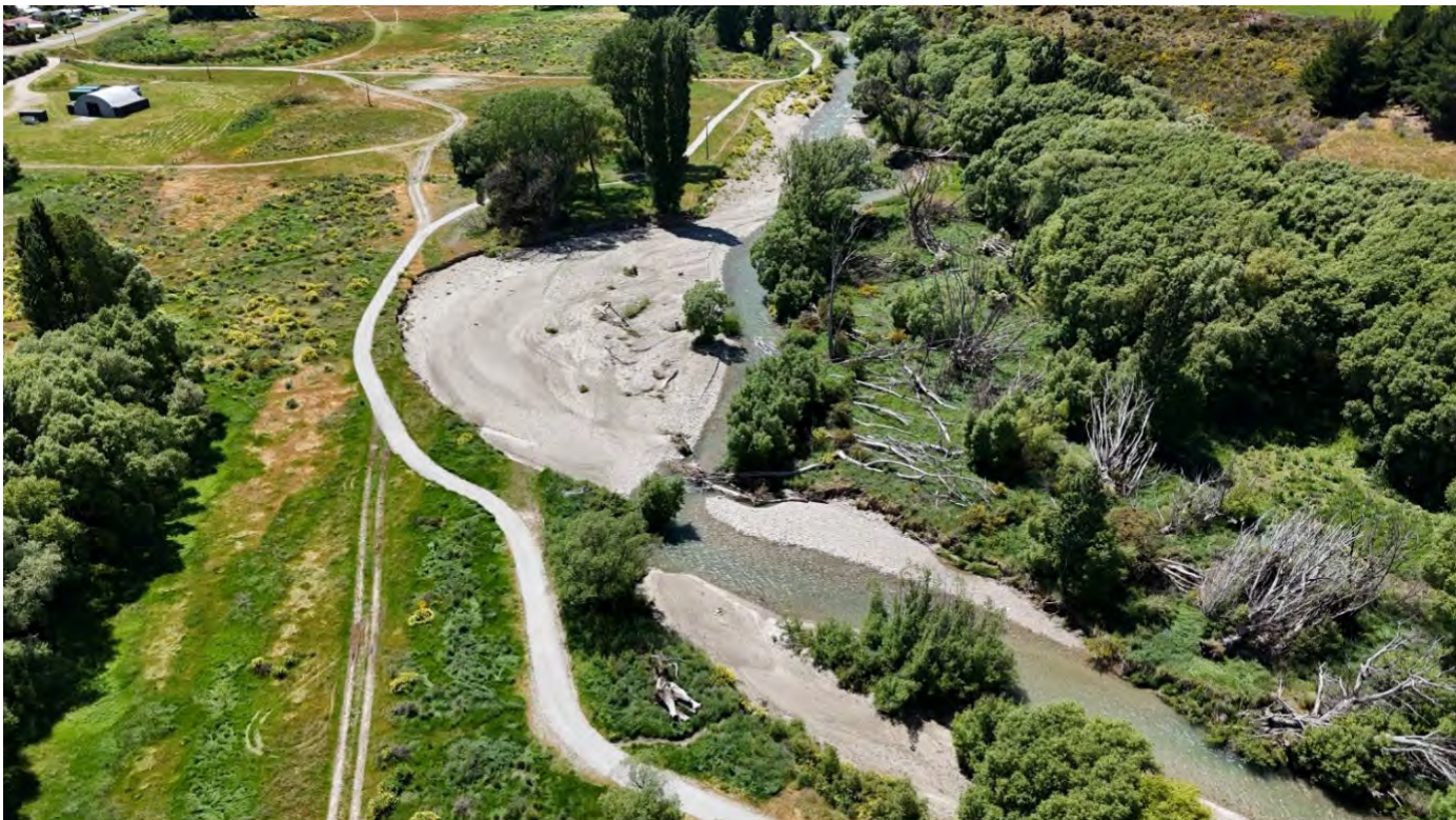
Figure 3. Aerial image of the bite that occurred during the event and encroaching on the road.
