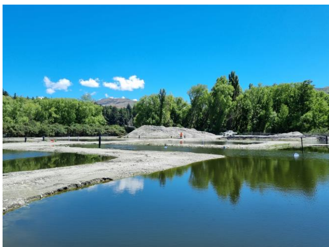
Figure 10 A portion of the existing disposal field, November 2024.
