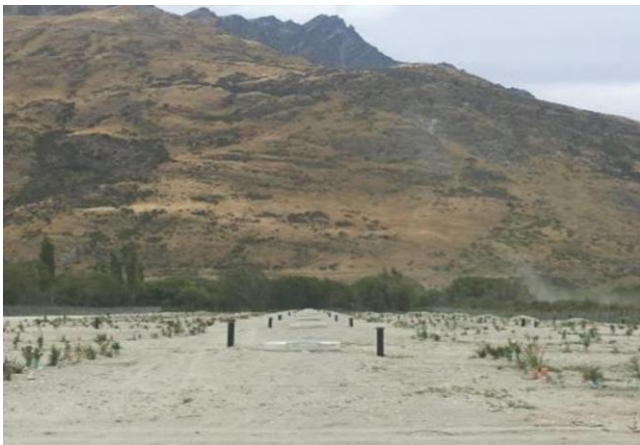
Figure 1 Disposal field post construction in 2019, photo provided by QLDC.
