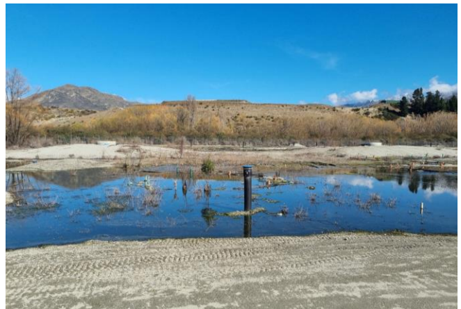
Figure 2 Disposal field ponding occurring in 2021 (although mounding/ponding was first observed in 2019), photo provided by QLDC.
