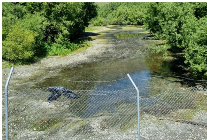
Figure 13 Surface runoff and ponding near the location of the disposal field, in a public area, November 2024.
