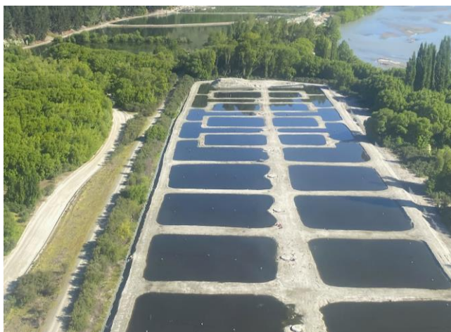
Figure 12 Existing disposal field, taken from above, November 2024.
