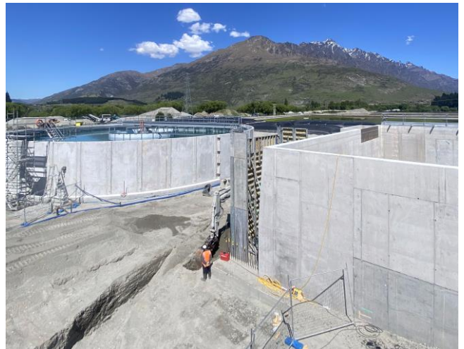
Figure 9 Stage 3 upgrades underway, November 2024.
