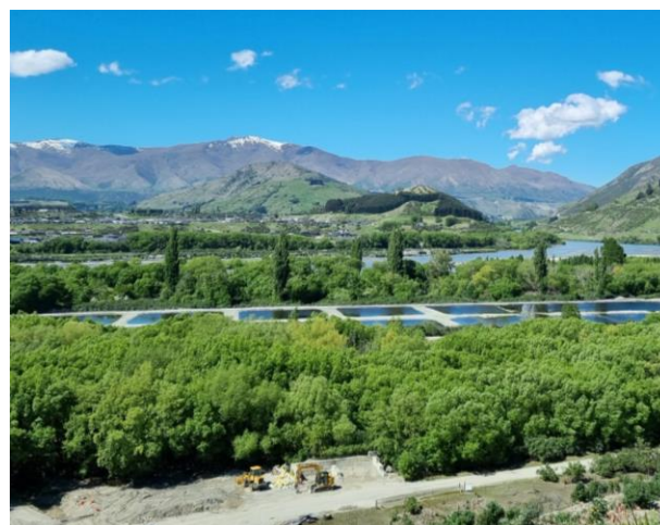
Figure 11 Existing disposal field, November 2024.
