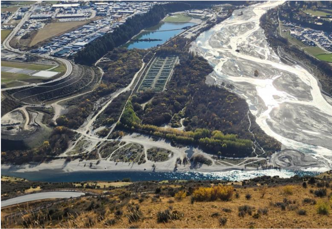
Figure 4. Photograph of the Site from the Remarkables Trig on 13 May 2026 showing existing vegetation cover along the proposed pipeline alignment (source: Dawn Palmer).
