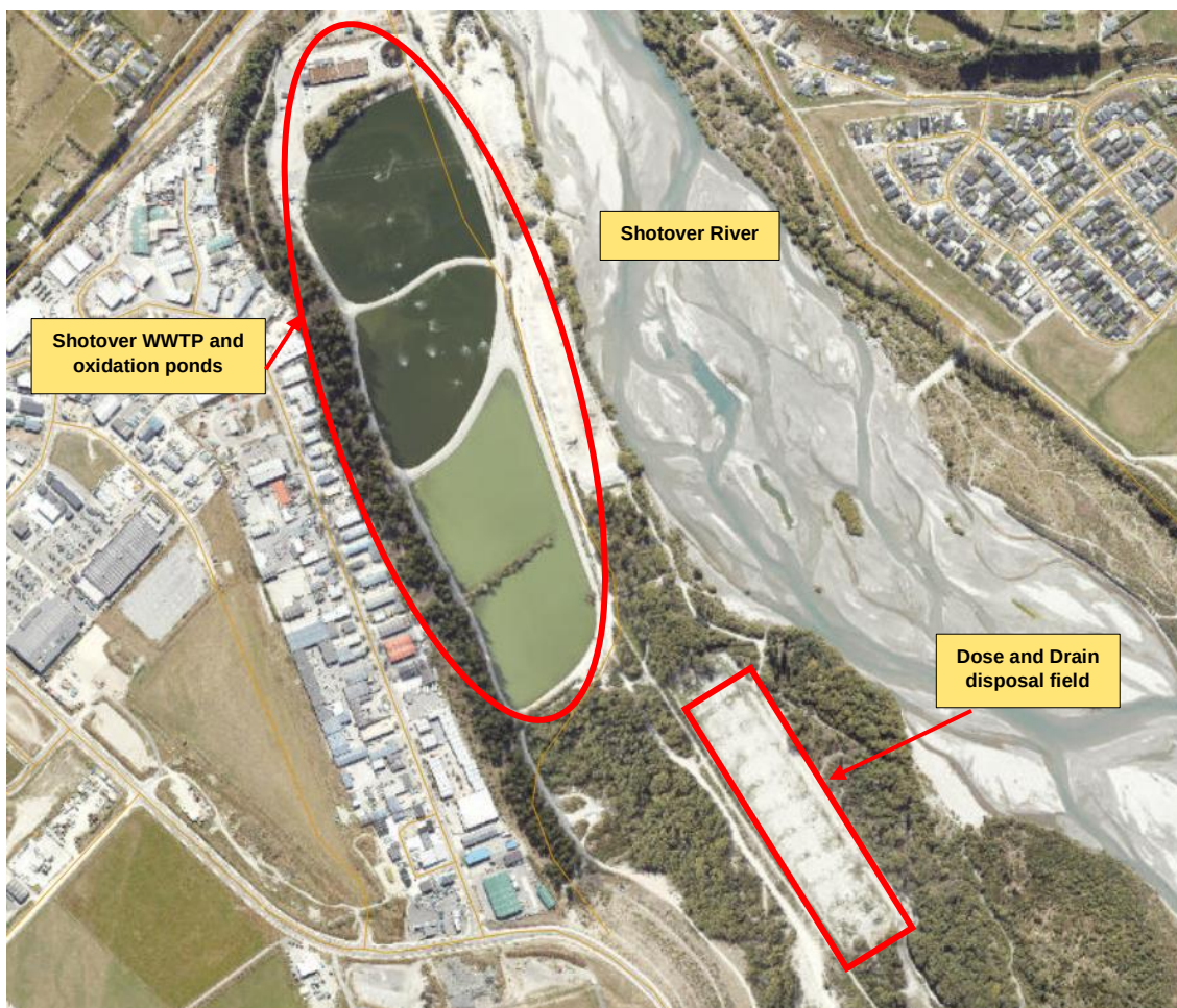
Figure 2-1: Aerial overview of the Shotover WWTP.
