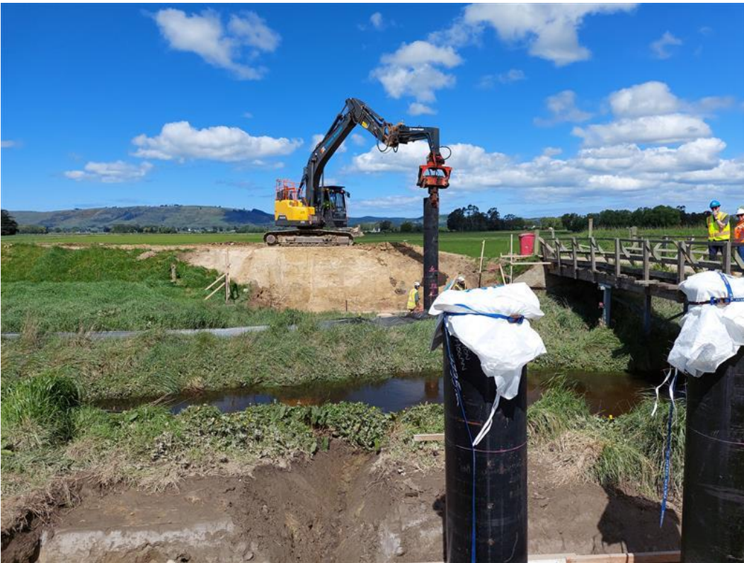
Figure 10 Bridge 14 site works underway
