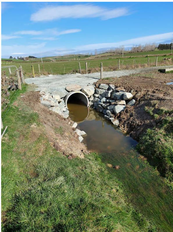
Figure 6 Toko Bridge 3 replaced with new culvert
