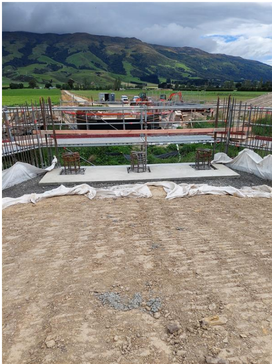
Figure 7 December 2024 Bridge 14 Headwalls almost complete
