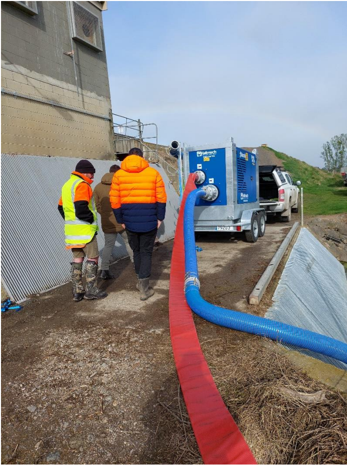
Figure 9 October 2024 New pump being tested at Silverstream
