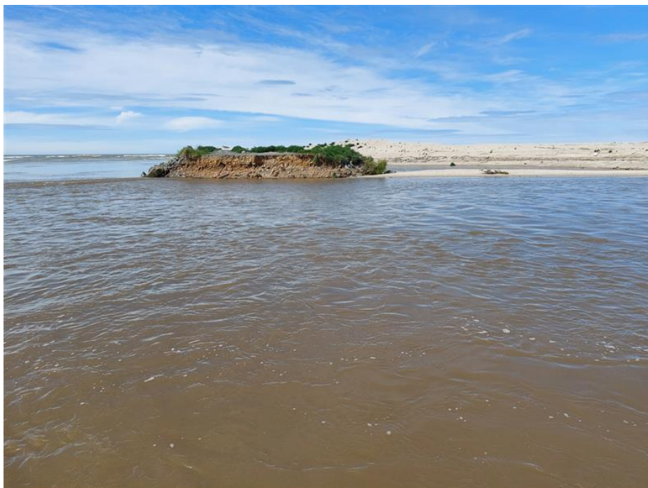
Figure 8 October 2024 Puerua Outfall damage visit after October rain event.
