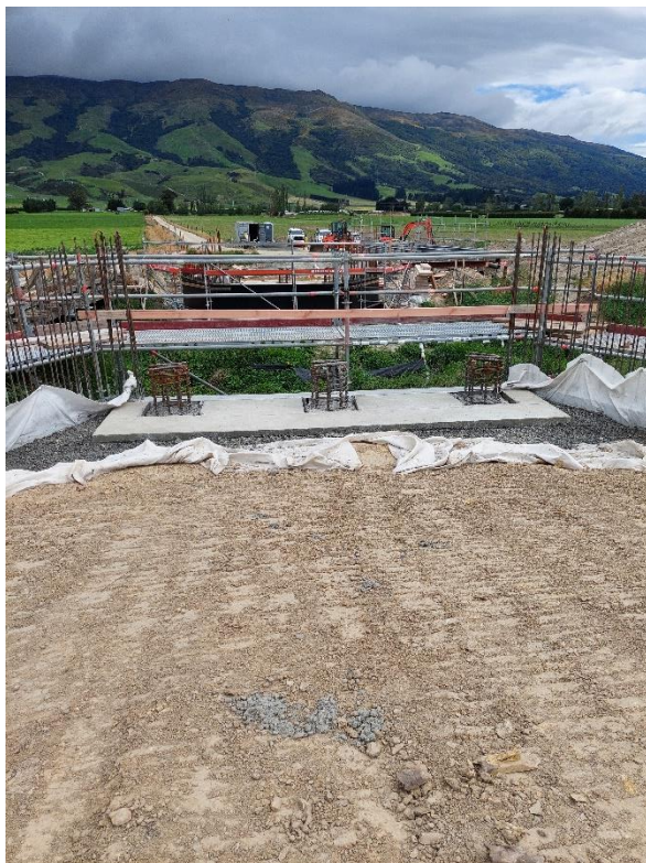
Figure 8 Climate Resilience Project: Bridge 14 headwalls almost complete.
