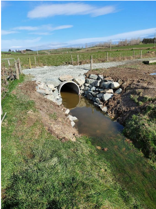
Figure 7 Climate Resilience Project: Toko Bridge, replaced with new culvert
