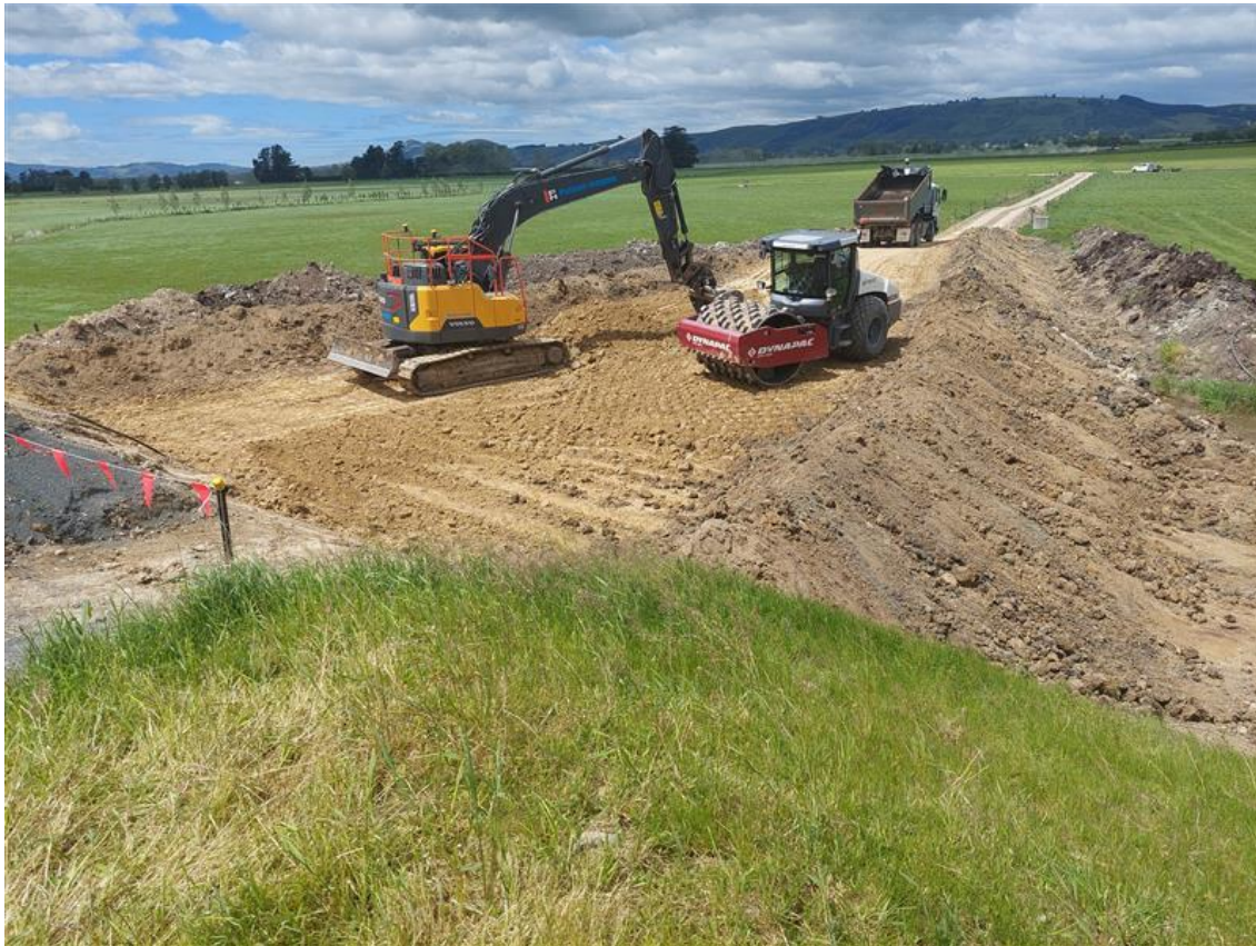
Figure 8 Bridge 14 approach road in construction
