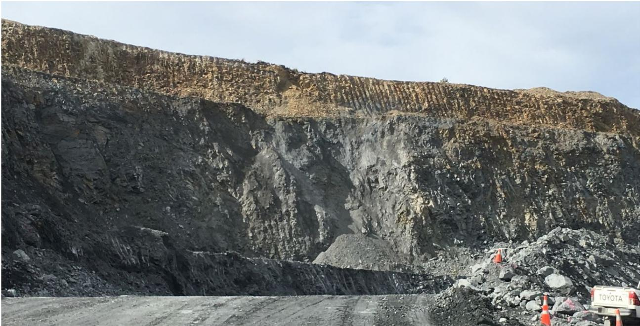
**Photo 5:** Coronation Pit Stage 2 – eastern wall of the ‘southern limb’. The 22.5 m high batters have not performed well in this rock mass.
