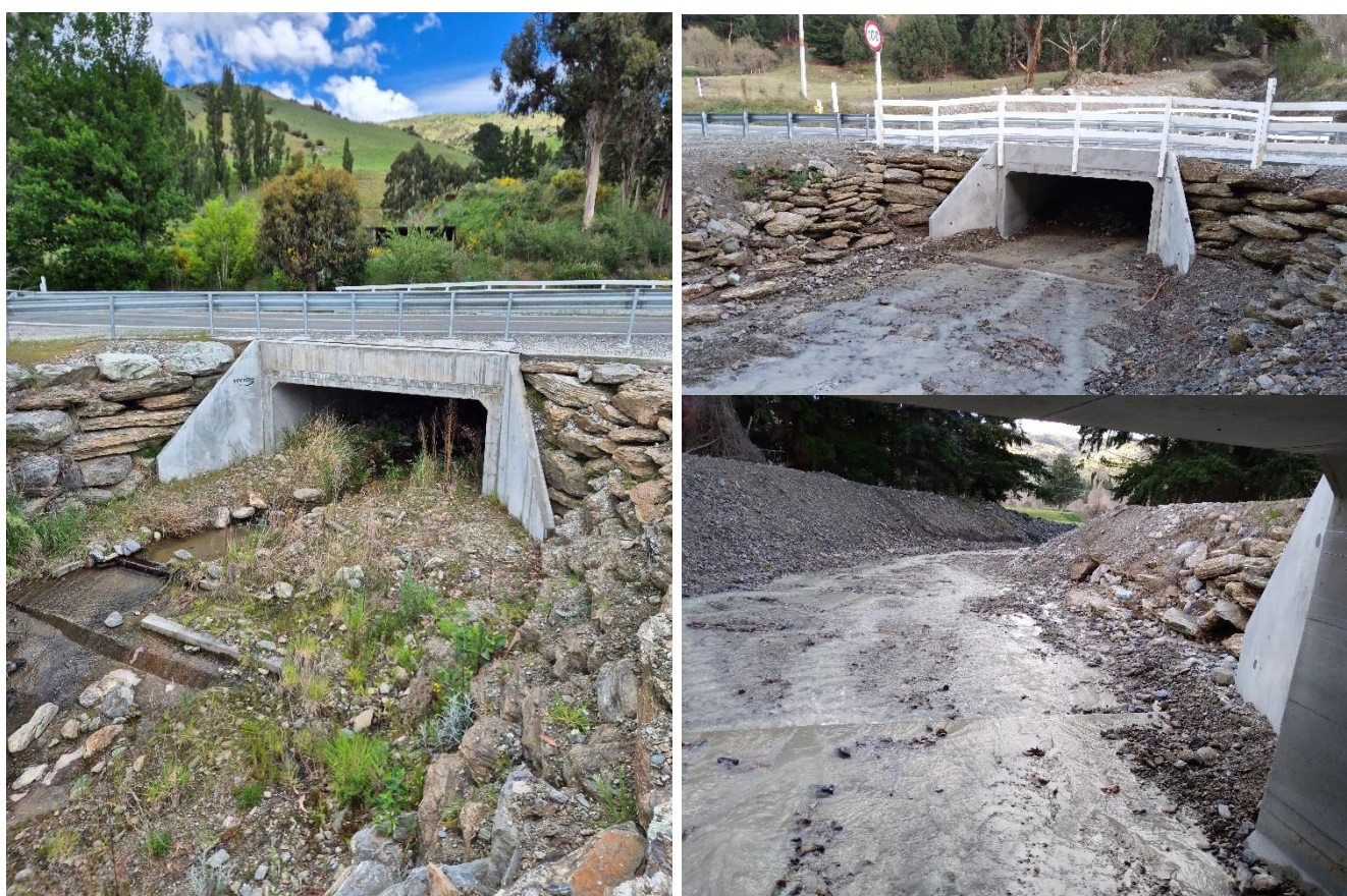
Figure 15: Culverts upgrades and channel works undertaken in Pumpstation (left) and Golfcourse Creek (right top and bottom). Left image was taken in early 2026 while the right two images were taken in 2023 during WSP fieldwork.
