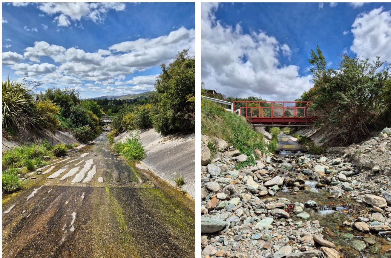
Figure 14: The concrete-lined chute at Reservoir Creek installed in the late 70's pictured here in early 2026 during WSP fieldwork.
