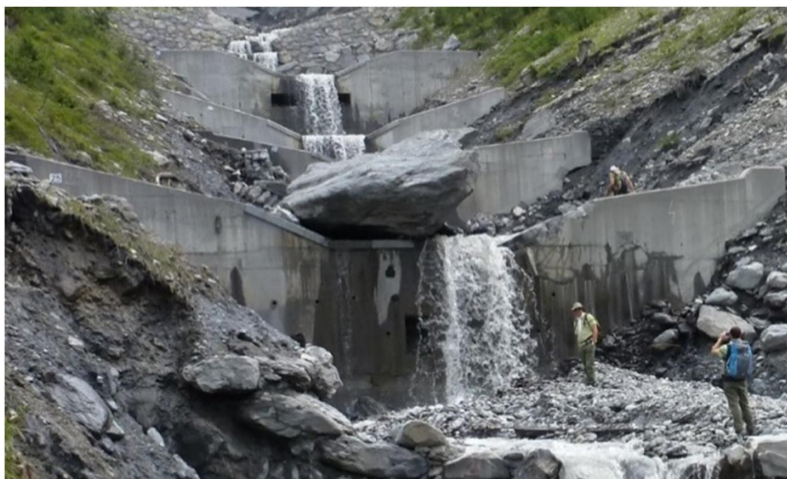
Figure 5: A cascade of check dams in the St Antione torrent upper basin (Piton G. , et al., 2017).
