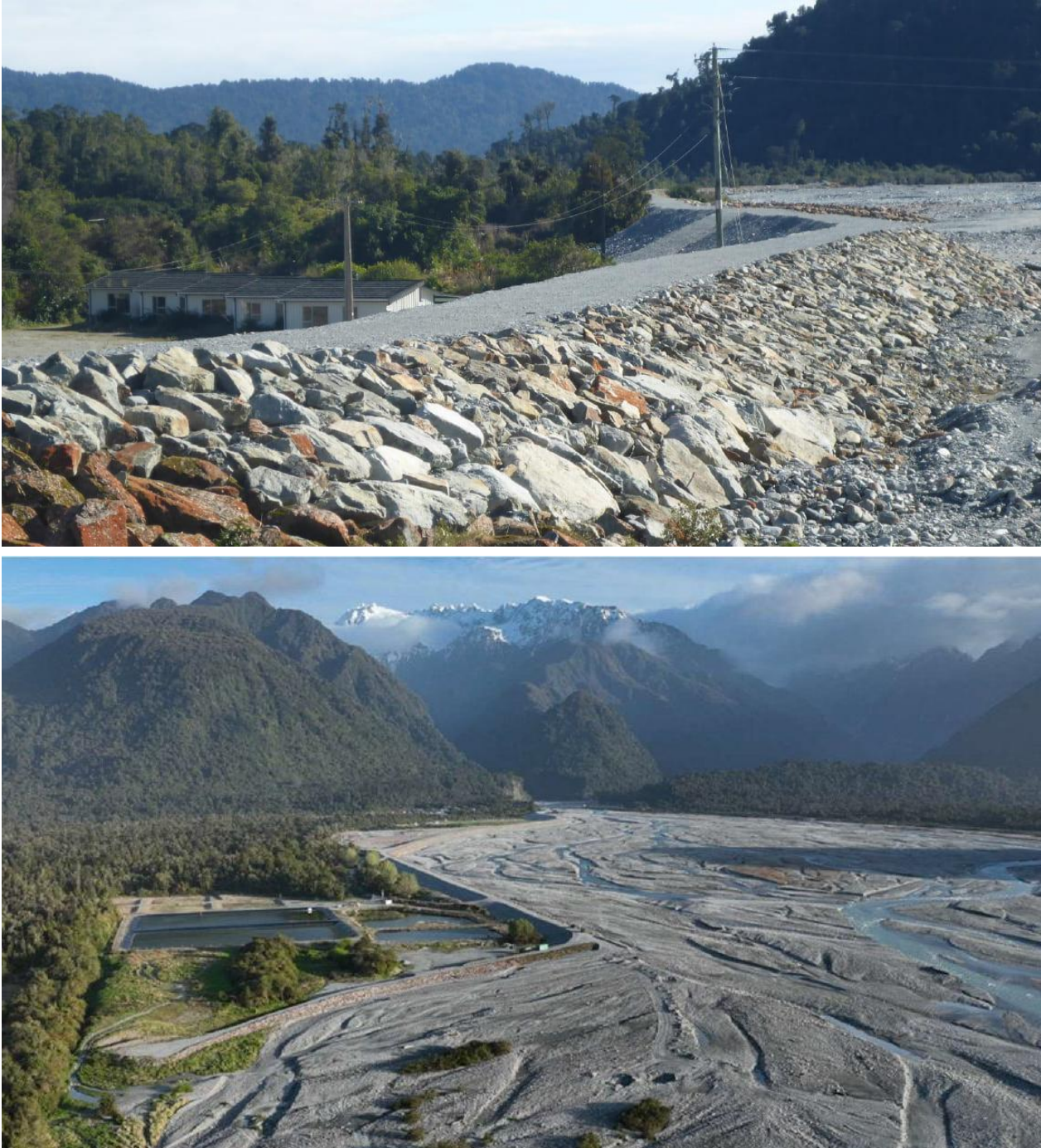
Figure 3: Stopbanks along the Waiho River in Franz Josef, New Zealand and exposed infrastructure built on the exposed floodplain. Top: A stopbank with disused motel units built at original fan level (University of Canterbury). Bottom: The waste water treatment plant at Franz Josef currently protected with engineered stopbanks (Otago Daily Times).
