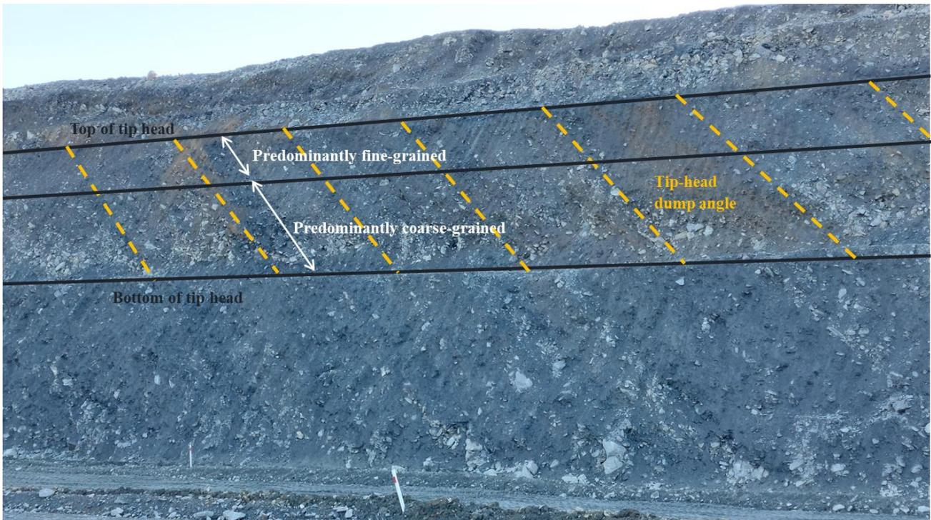
Figure 7.2 Waste rock segregation from tip head dumping (from historic backfill at the IM6 cut face)
