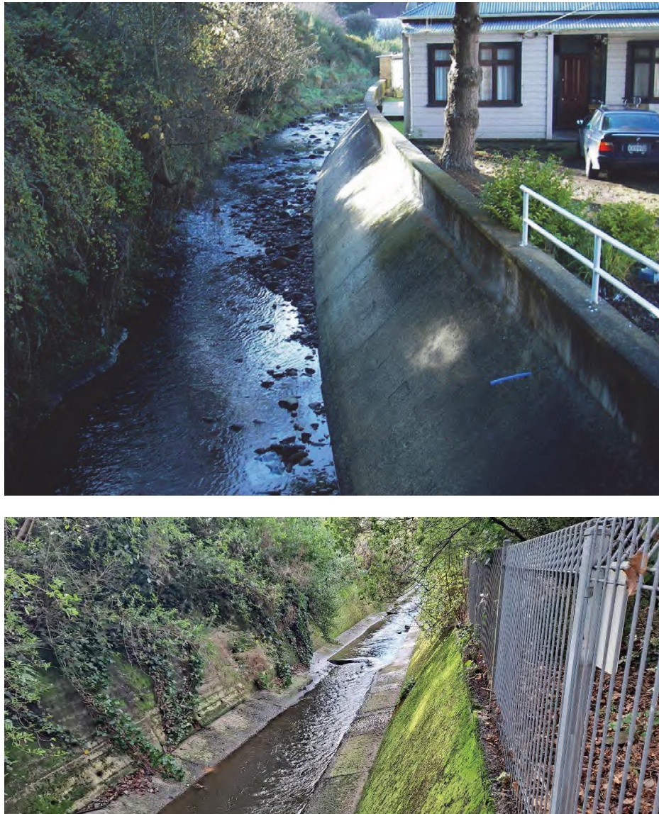
Figure 2. Typical sections of the Lindsay Creek channel in North East Valley (all looking upstream). Note the narrowness of the channel, the steepness of the right bank and the proximity of the houses and residential activities at many locations along the stream channel. The concrete channel lining and floodwall are ORC assets, some infrastructure is also owned, controlled and maintained by Dunedin City Council and adjacent private landowners.
