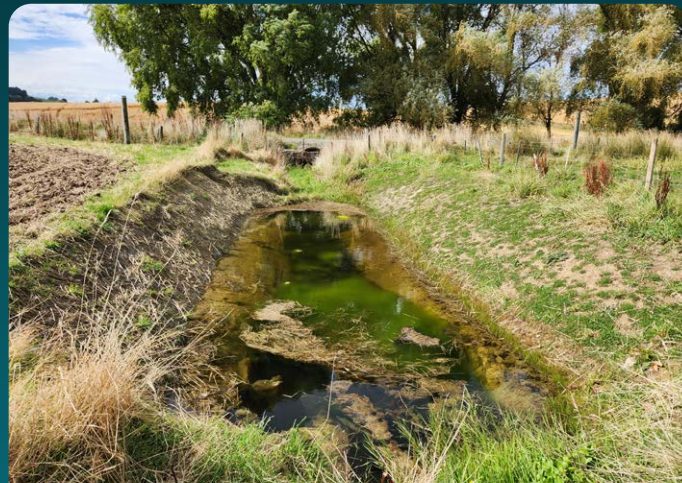
Figure 3. Example of a simple sediment trap that requires maintenance, located next to a paddock used the previous winter for grazing livestock.
