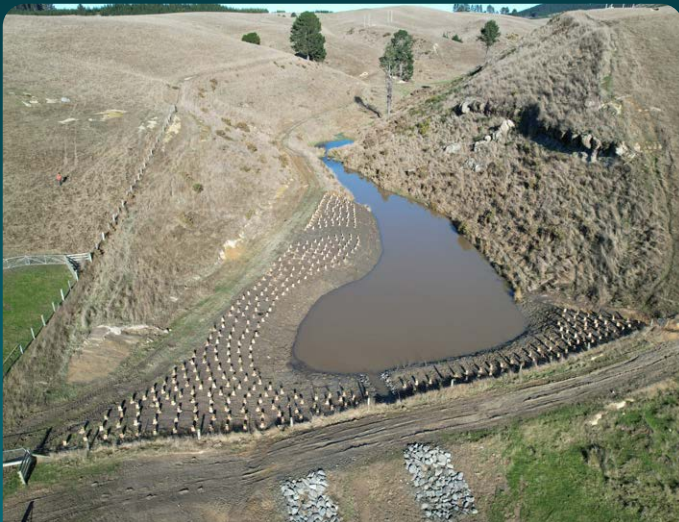
Figure 2. Example of a sediment trap recently constructed in East Otago.
