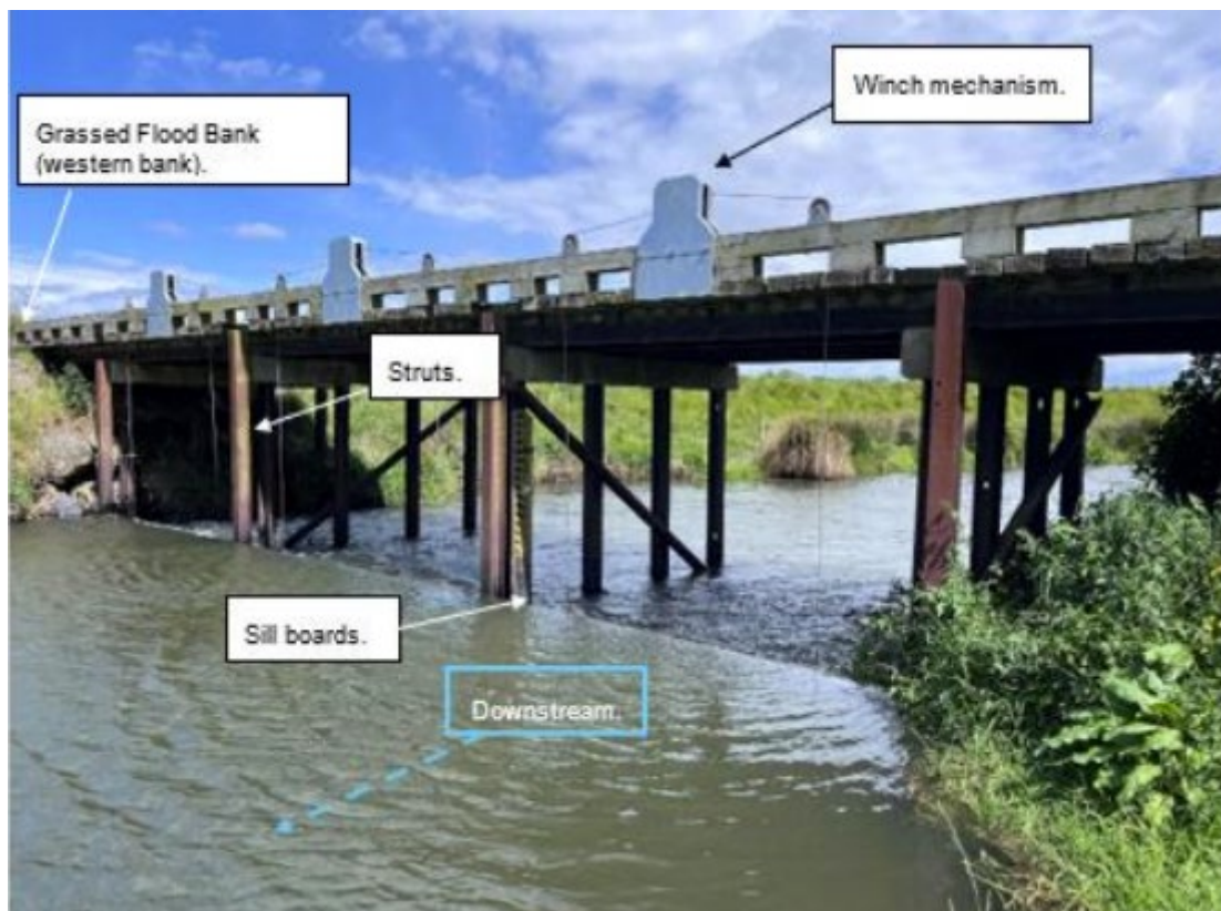
Figure 1: Current outlet sill structure (Source: Application)
